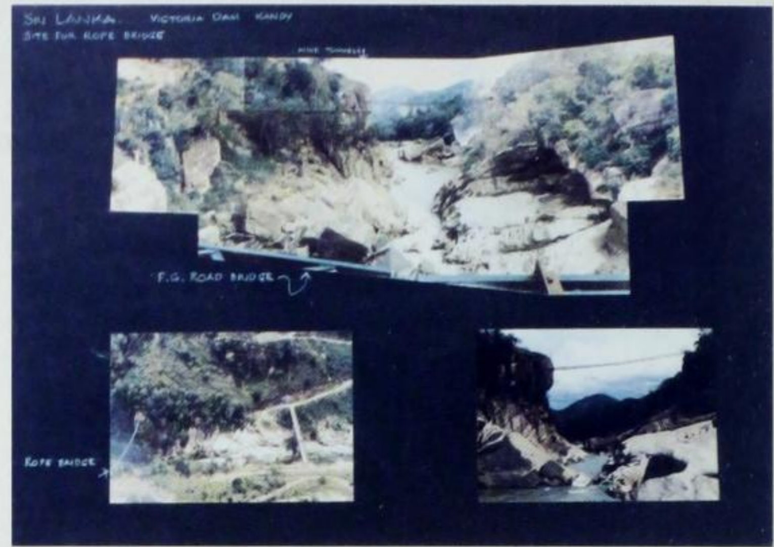
Site for rope bridge, photo collage, location work in Sri Lanka
