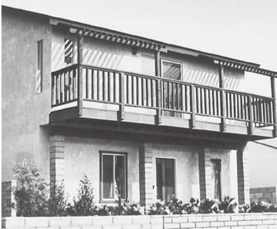
Figure 17-13. Typical uses of cantilevered framing.
