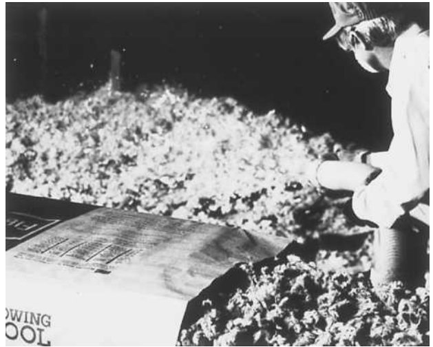
Figure 31-5. Blowing wool.
