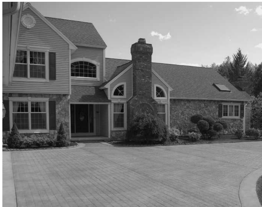
Figure 1–1(a). Single- and multi-family homes are classified as residential construction.
