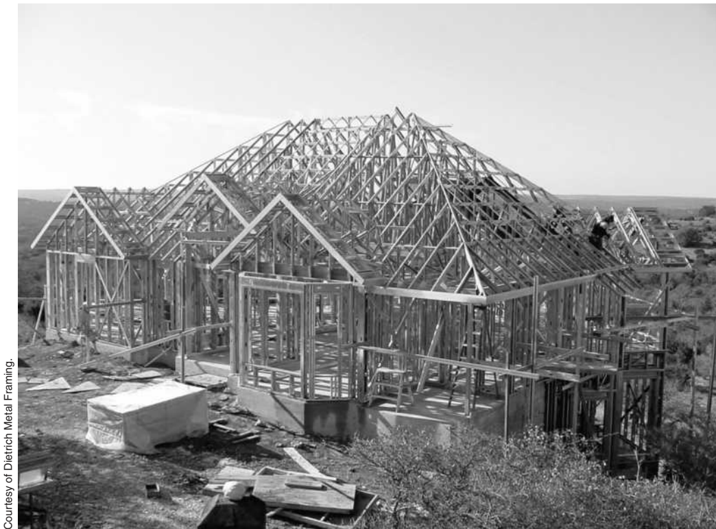
Figure 15–15. Metal framing.
