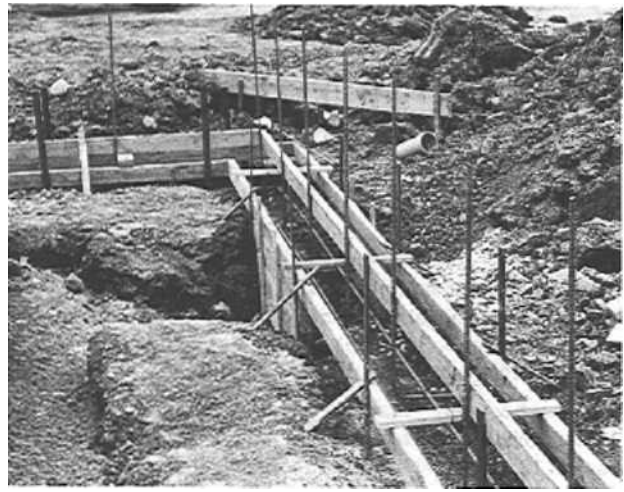
Figure 12-6. Footing forms.
