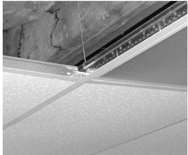
Figure 31-8. Suspended ceiling.
