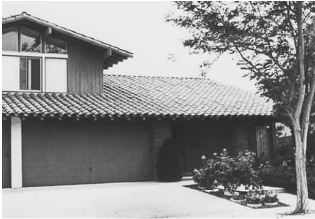
Figure 22-5. Tile roofs are popular in some parts of the country.
