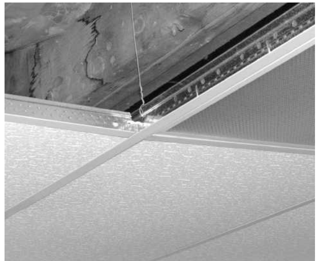
Figure 31-8. Suspended ceiling.
