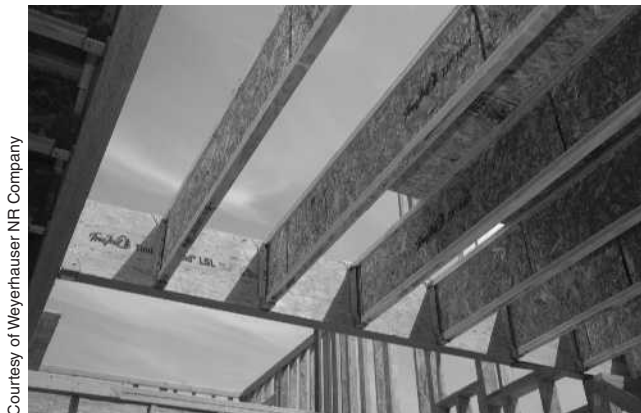
Figure 17-5. When I-joists are used for floor framing, the joist header is usually an engineered rim board.
