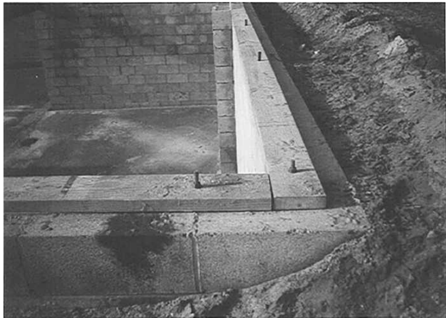
Figure 17-1. Sill plate.
