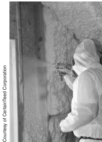
Figure 31–2. Foamed-in-place insulation.
