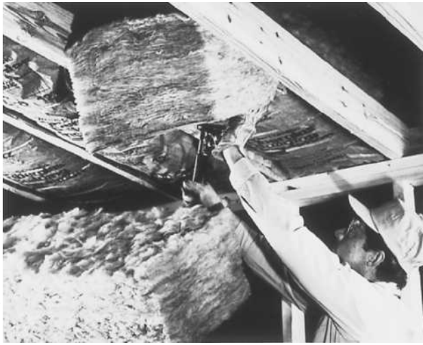
Figure 31-4. Blanket insulation.
