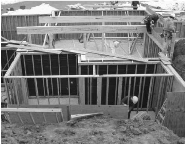
Figure 13–9. Permanent wood foundation.
