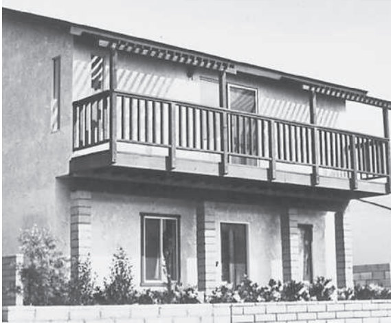
Figure 17-13. Typical uses of cantilevered framing.
