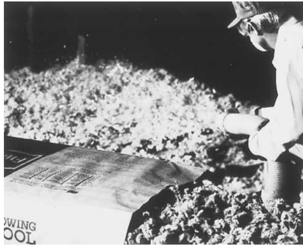
Figure 31-5. Blowing wool.
