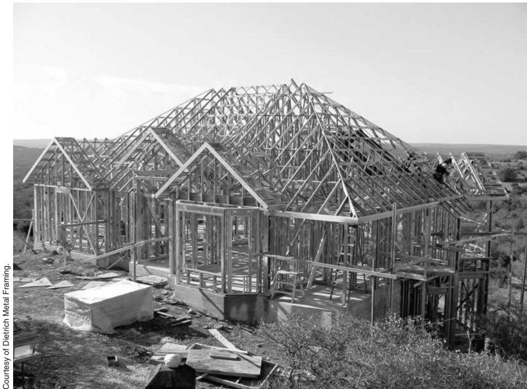
Figure 15–15. Metal framing.
