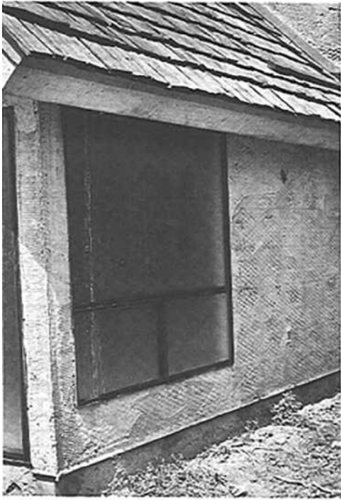
Figure 26–12. Scratch coat applied.
