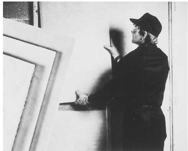
Figure 31–3. Rigid insulation.
