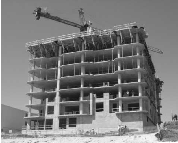
Figure 1–1(b). Commercial construction.
