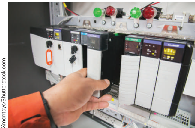
FIGURE 10-6 A technician removing a module from the rack. Notice how it comes out straight because of the guide rails built into the rack as well as the ventilated metal on top.
