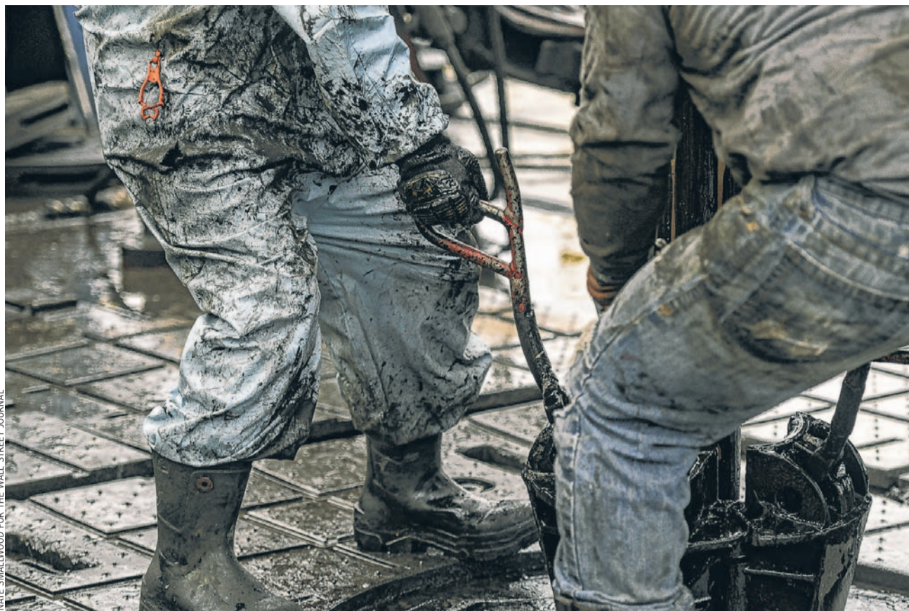
Drilling work at a Range Resources site in Pennsylvania. The natural-gas producer aims to build a well 25,000 feet in length.
