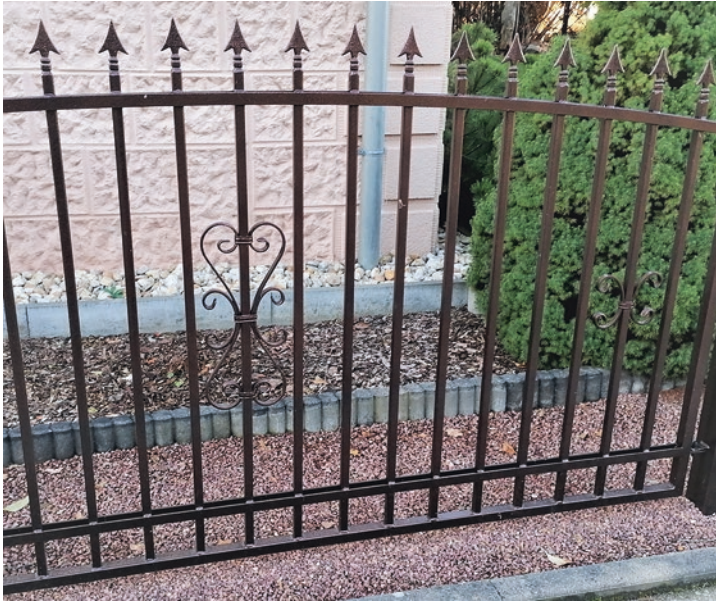
Fig. 2.9 Garden fence made of forged iron, painted to protect against corrosion. (Photo: Schlegel, J.)
