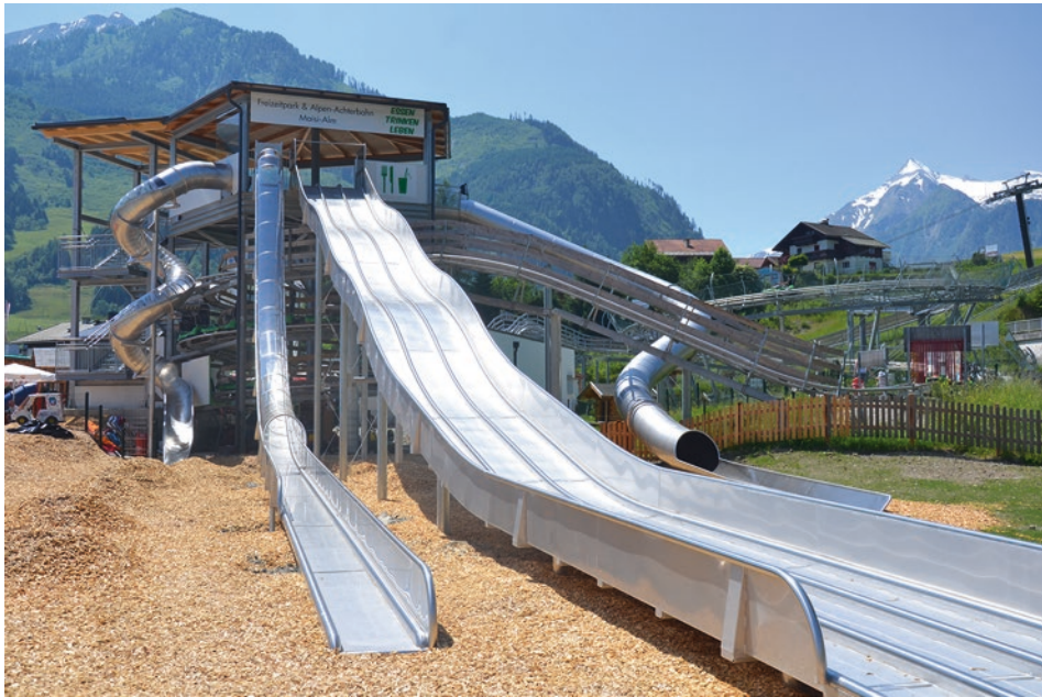
Fig. 11.10 Attractions made of stainless steel in a leisure park. (Photo: Josef Wiegand GmbH & Co. KG, Rasdorf)
