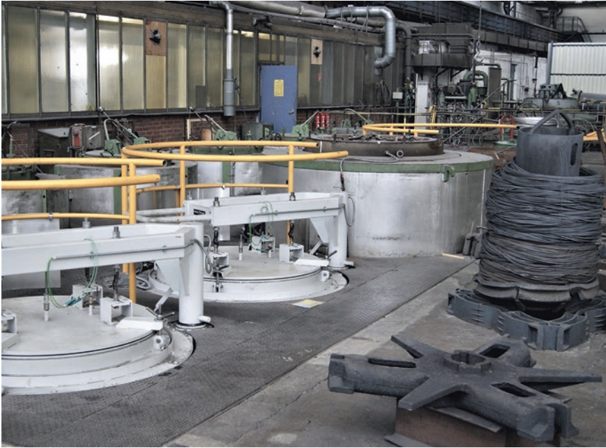
Fig. 6.16 Pot annealing furnaces for annealing of drawn wire. (Photo: Schlegel, J., BGH Edelstahl Lugau GmbH)
