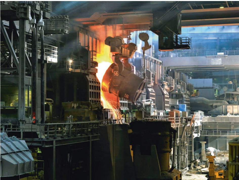
Fig. 4.12 View of the Thyssenkrupp Steel Europe AG oxygen steel mill in Duisburg. (Photo: Thyssenkrupp Steel Europe AG)
