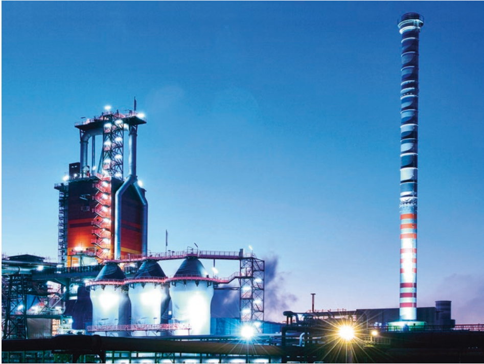
Fig. 4.7 View of blast furnace 8 of Thyssenkrupp Steel Europe AG in Duisburg. (Photo: Thyssenkrupp Steel Europe AG)
