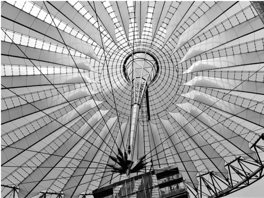
Fig. 1.3 Steel roofing structure of the Sony Center at Potsdamer Platz, Berlin. (Photo: Schlegel, J.)
