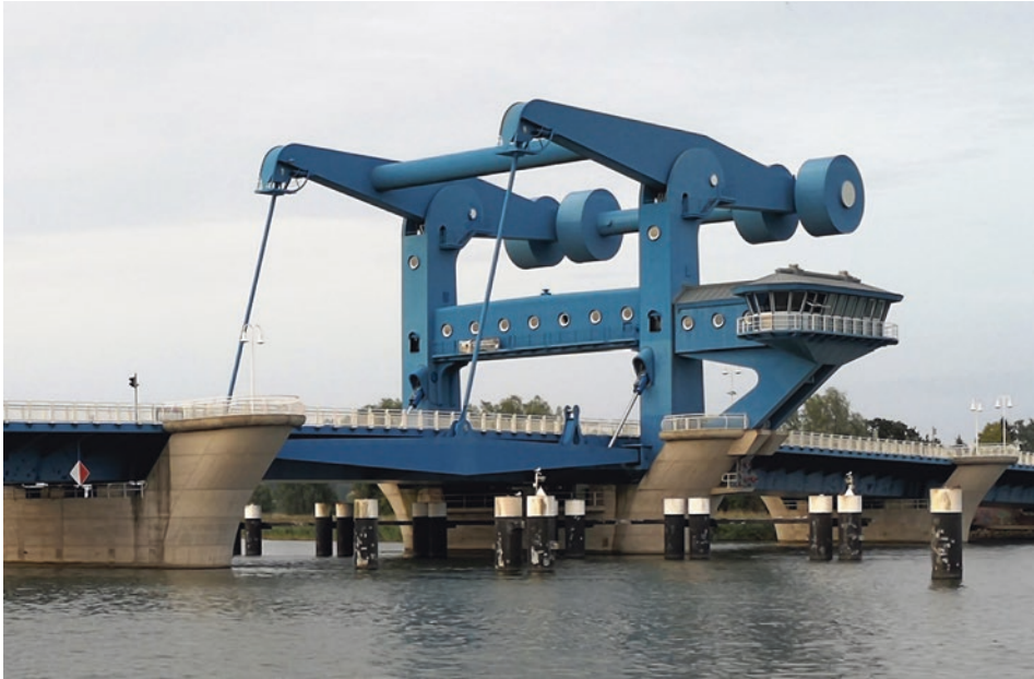
Fig. 2.15 Peenebrücke in Wolgast. (Photo: Schlegel, J.)
