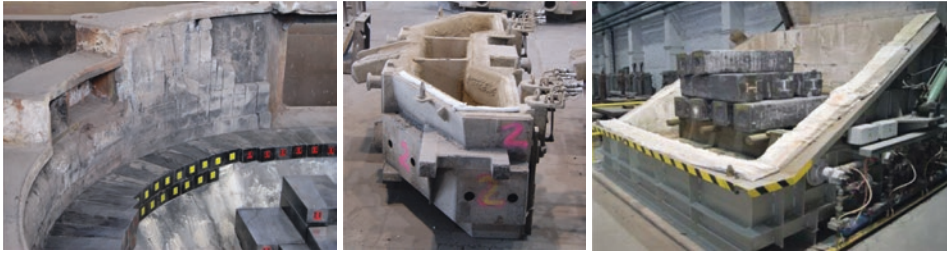
Fig. 10.10 New refractory linings from left to right : melting vessel of an electric arc furnace, distributor for a continuous casting plant, pot annealing furnace. (Photos: Schlegel, J., BGH Edelmetall Freital GmbH)
