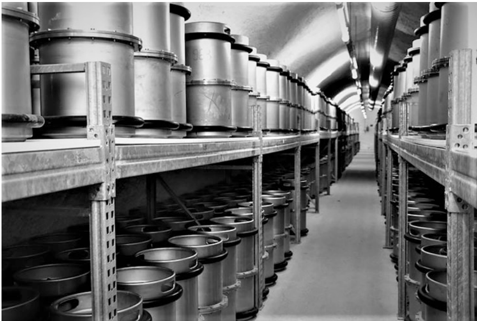
Fig. 11.1 Barbara Tunnel with stored stainless steel barrels. (Photo: Straube, B., BBK – Federal Office for Civil Protection and Disaster Assistance, Bonn)
