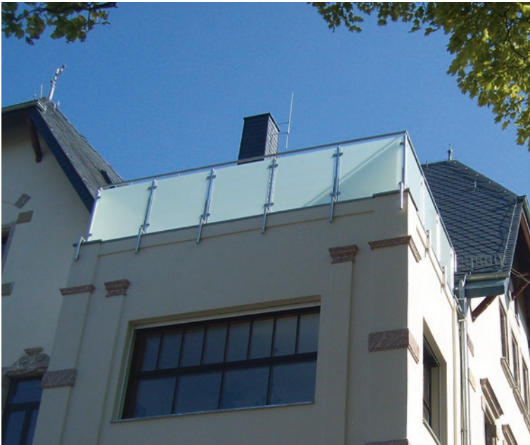
Fig. 11.2 Parapet on a balcony with handrail and posts made of stainless steel 1.4301 - X5CrNi18-10. (Photo: Strzelczyk, R., Strzelczyk Edelstahl-Verarbeitung, Rossau)
