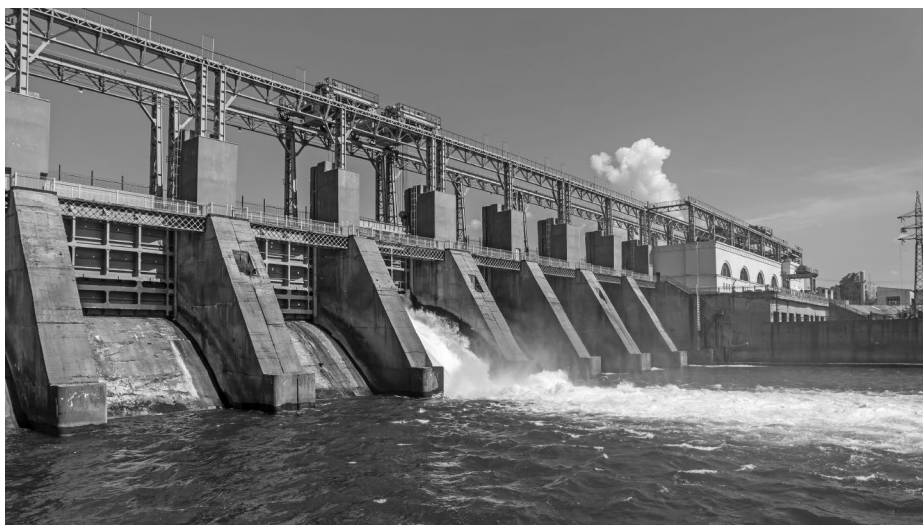
Hydroelectric generating stations produce electricity important for industry and residence areas. Maxim Burkovskiy/Shutterstock
