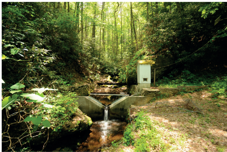
Box Figure 1.1a An example of an experimental weir for hydrological and hydrochemical monitoring in an experimental catchment at Coweeta.
