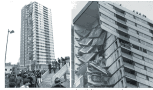
(c) Ronan Point building, London, collapsed in 1968, gas explosion [16]
