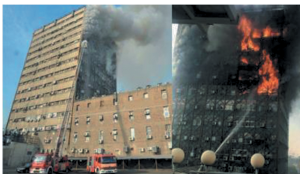
(m) Plasco tower in Iran, collapsed in 2017, fire [25]
