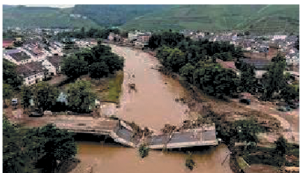
(p) Bridge collapse in Bad Neuenahr-Ahrweiler, Germany, 2021, flood [28]
