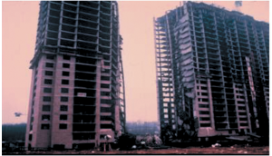
(d) Skyline Plaza in the USA, collapsed in 1973, framework removal [17]
