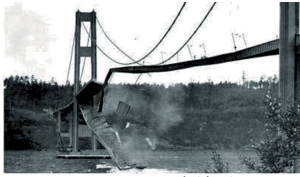
(a) Tacoma Narrows bridge in Washington, collapsed in 1940, wind [14]
