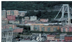
(n) Morandi bridge in Italy, collapsed in 2018, poor construction [26]
