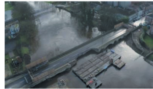
(l) Tadcaster bridge in England, collapsed in 2015, river scour [23,24]
