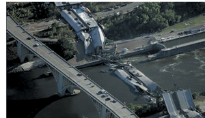
(i) I-35W bridge in Minneapolis, USA, collapsed in 2007, design flaw [21]
