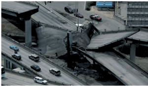
(j) I-580 Connector Ramp –Oakland, California, collapsed in 2007, fire [18]
