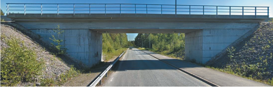
Figure 5.7: Hörnefors railway bridge.
