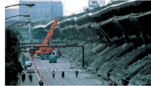
(f) Hanshin Expressway bridge in Kobe, Japan, collapsed in 1995, earthquake [19]
