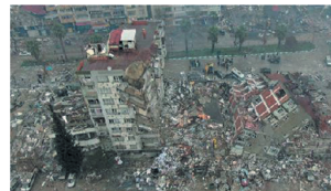
(r) Building collapse in Kahramanmaraş, Turkey, 2023, earthquake [31]
