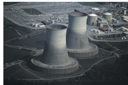
The Sequoyah Nuclear Power Plant in Tennessee uses water to transform nuclear energy into electrical energy. Brand X Pictures/Alamy Stock Photo
