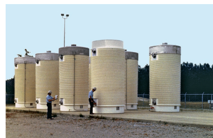
Figure 9.9 These storage tanks are designed for radioactive waste. Source: U.S. Nuclear Regulatory Commission
