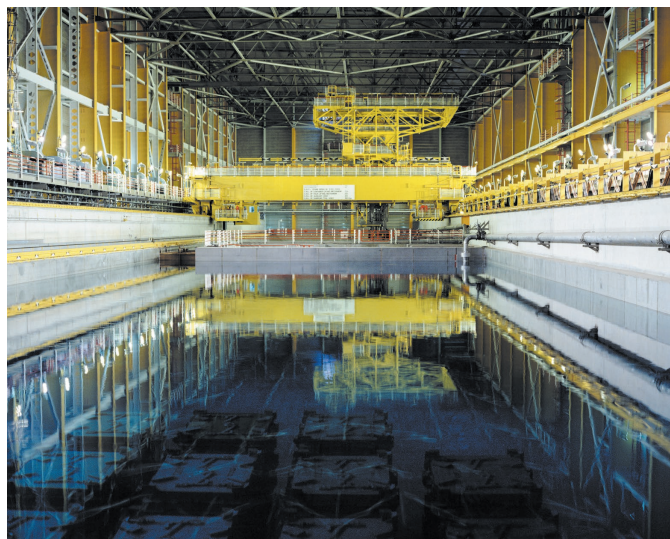
Spent nuclear fuel is temporarily stored in a storage pond. Steve Allen/Brand X Pictures/Alamy Stock Photo
