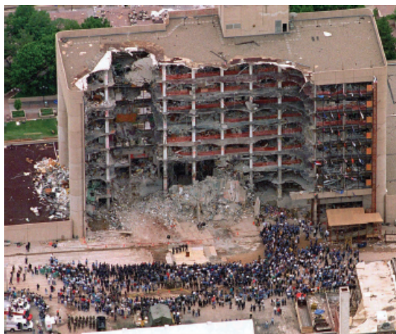
The Alfred P. Murrah building after a deadly explosion caused by an ammonium nitrate bomb.
