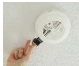
A smoke detector sounds an alarm when smoke enters its ionization chamber.
