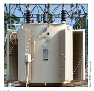
**FIGURE 28–43** Three-phase autotransformer.
