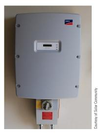
**FIGURE OCCUPATIONS 5** Inverter changes the direct current produced by the solar cells into alternating current.
