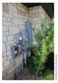
**FIGURE OCCUPATIONS 6** One meter records the power supplied by the utility company, and another records the amount of power supplied by the solar panels.
