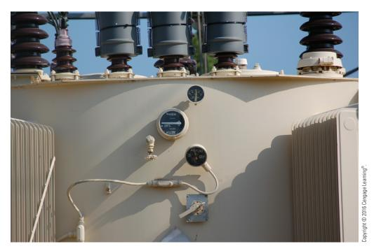
FIGURE 29-4 External gauges used to monitor a sealed transformer.
