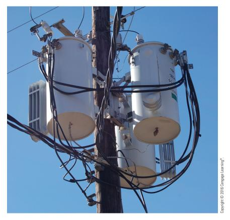
**FIGURE 29–7** Three single-phase transformers connected to form a three-phase bank.
