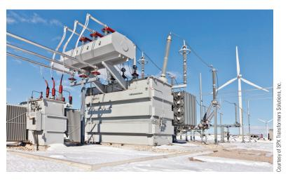
FIGURE 29–3 Pad-mounted transformer with dry nitrogen bottle.
