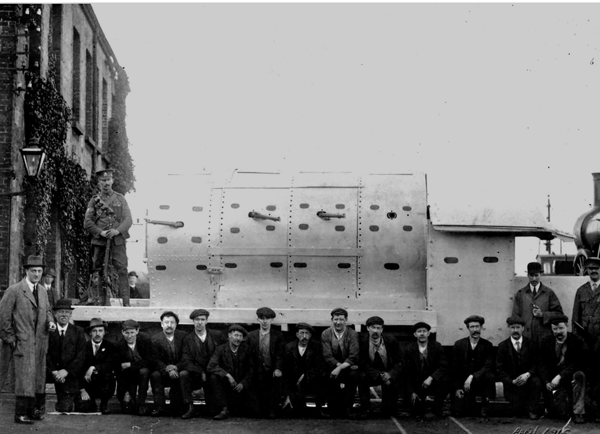
ARMoured VEHICLES MADE FROM LOCOMOTIVE SMOKEBOXES ON LORRIES; 1916 INCHICORE
