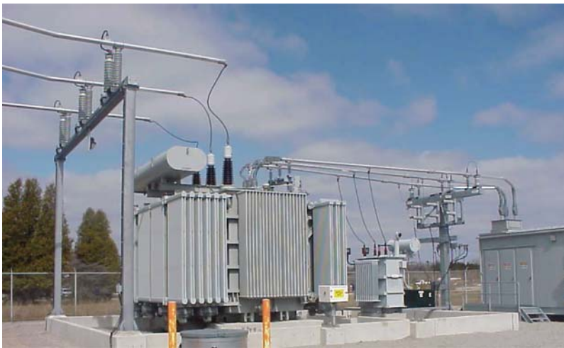
Figure 5.1 (a) An example of a single-line diagram. (b) An example actual station (partial) for the single-line diagram.
