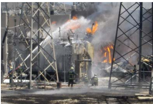
Figure 1.3 Failed transformer on fire – Thessaloniki Greece. Source: Konstantinos Stampoulis / Firefighters.gr / Wikimedia Commons / CC BY-SA 3.0 GR.
