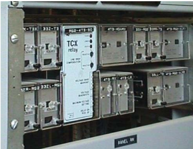
Figure 2.7 Mounting of legacy auxiliary logic.
