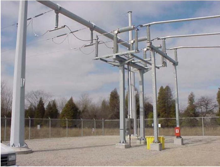
Figure 10.10 S&C Series 2000 115 kV circuit switcher and disconnect. Source: Photo Courtesy of S&C Electric Co.
