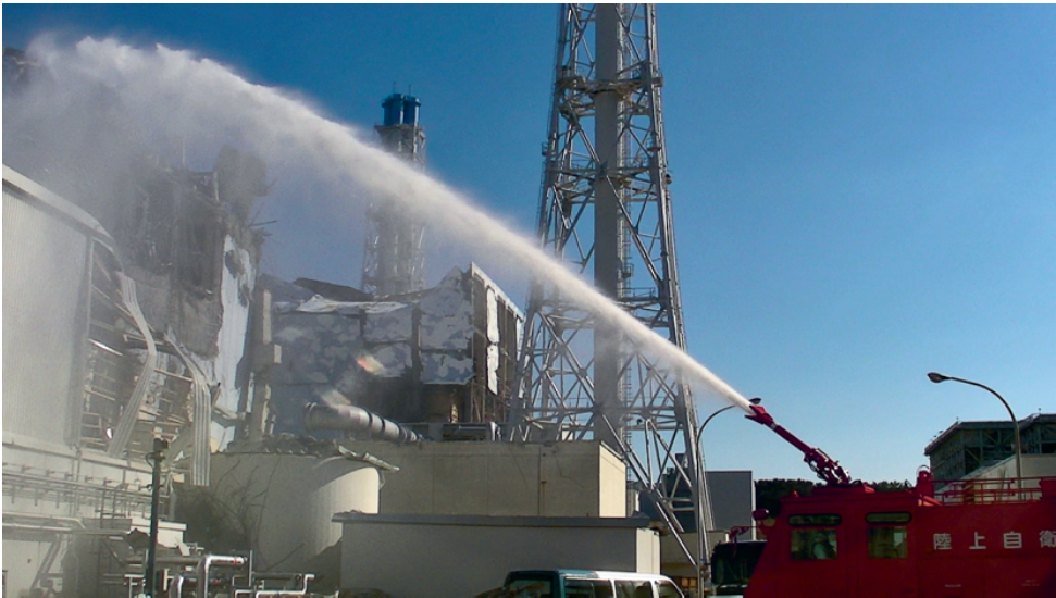
Figure 4. Fire at a power plant in Fukushima Daiichi, Japan, in March 2011. The various engine failures due to the tsunami caused the breakdown of the cooling system of the reactor. The intense heat produced by the fission reaction induces chemical reactions leading to the decomposition of the cooling water with the emission of hydrogen. This hydrogen then exploded, and radioactive products were emitted in the atmosphere.
