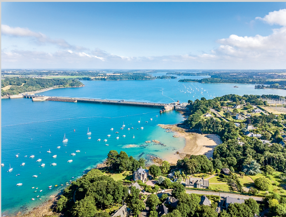
In Northern France (the Bretagne), this tidal barrage on the river Rance has been operating since 1967. The barrage, which also serves as a bridge,
