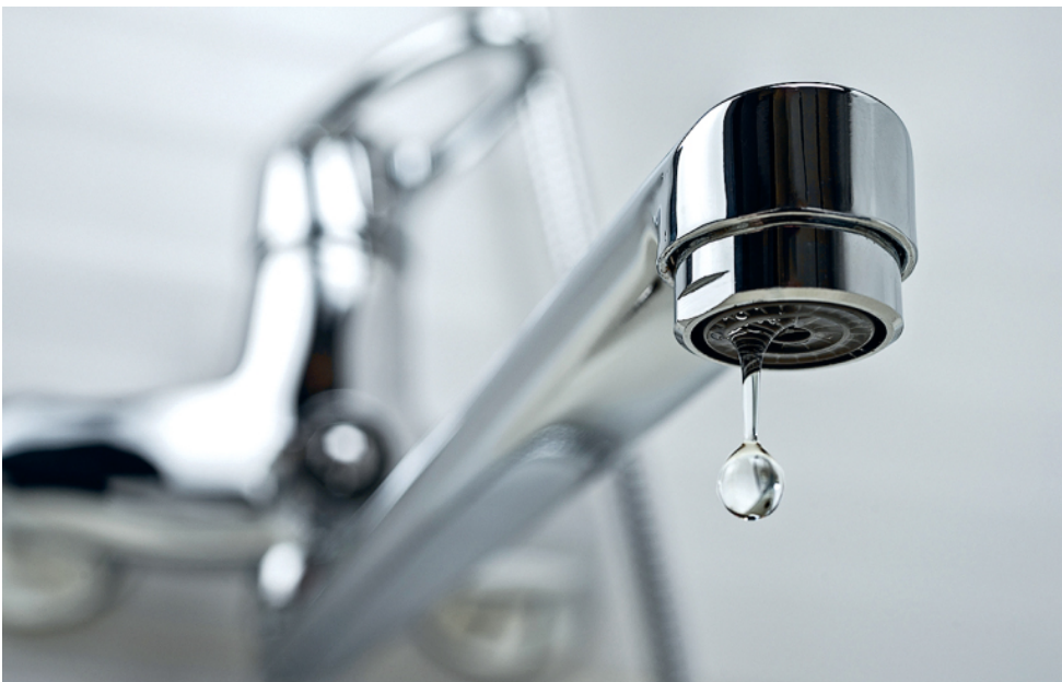
Figure 11. A badly fitted tap lets drops fall. The dynamics of the formation of the drops is complex and was studied in detail during the 1990s.
