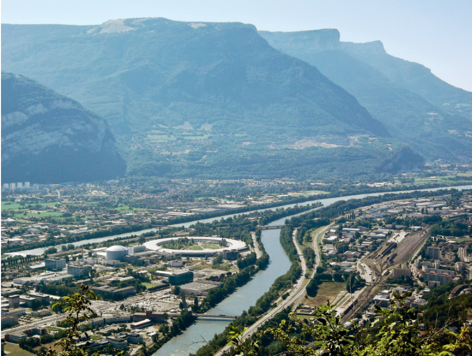
Figure 4. The ESRF synchrotron ring at the confluence of the Isère (above) and Drac rivers. Electrons under the influence of a magnetic field move in a ring at a speed close to the speed of light. When the direction of speed changes, they emit intense X-rays. On the right in the cylindrical domed building is the nuclear reactor of the Laue-Langevin Institute.
