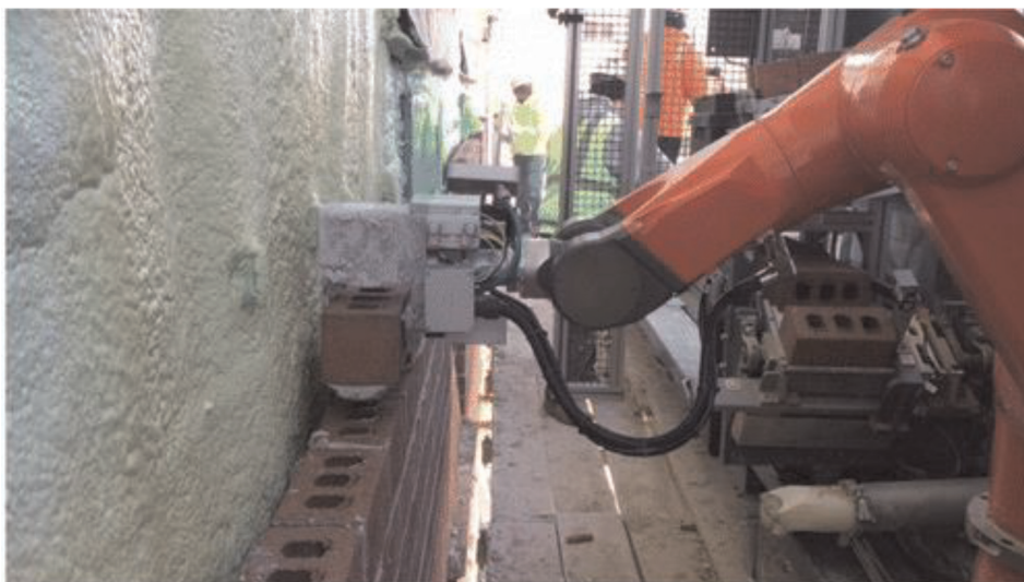
Figure 6. SAM100 robot onsite screenshot. Source: Podkaminer and Peters [45].
