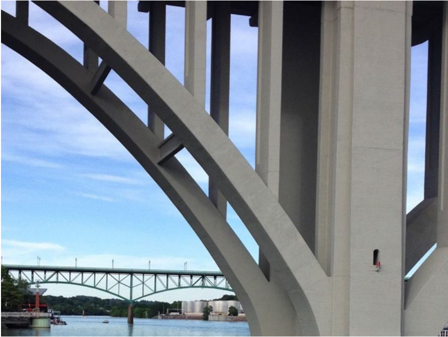
Figure 8-1. Two bridges in Knoxville, Tennessee
