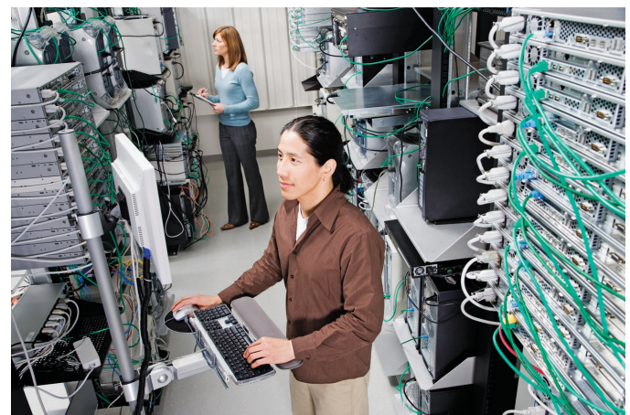
FIGURE 23.21 Computers make routine weather forecasts possible by solving mathematical equations that describe changes in a mathematical model of the atmosphere. Source: Fuse/Getty Images
