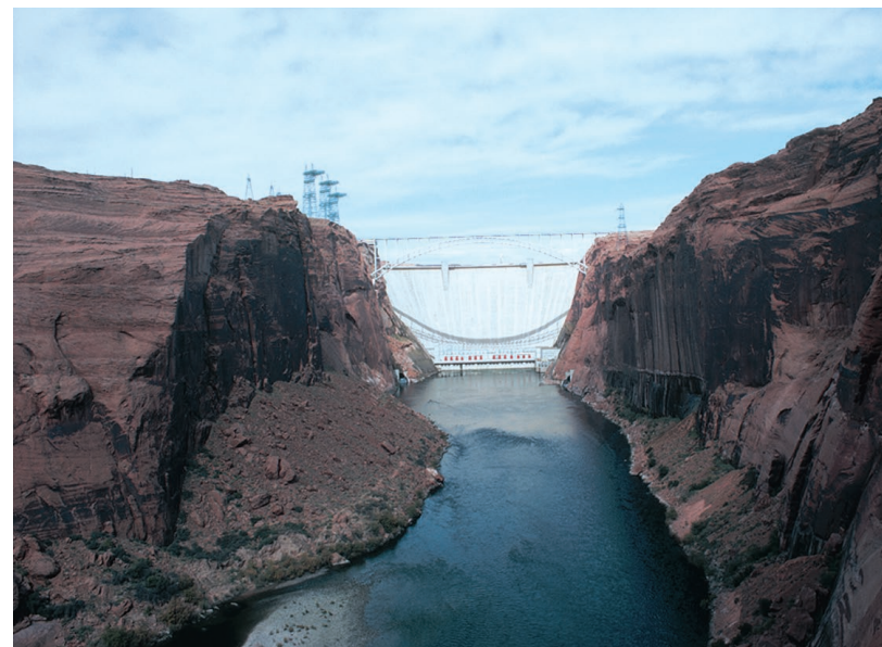
FIGURE 3.1 This is Glen Canyon Dam on the Colorado River between Utah and Arizona. The 216 m (about 710 ft) wall of concrete holds Lake Powell, which is 170 m (about 560 ft) deep at the dam when full. Water falls through 5 m (about 15 ft) diameter penstocks to generators at the bottom of the dam. ©McGraw-Hill Education/Bill Tillery, photographer
