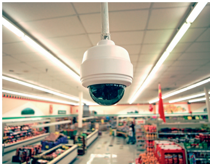
FIGURE 8.12 These long tubes of fluorescent lights emit light as electrons of mercury atoms inside the tubes gain energy from the electric current. As soon as they can, the electrons drop back to a lower-energy orbit, emitting photons with ultraviolet frequencies. Ultraviolet radiation strikes the fluorescent chemical coating inside the tube, stimulating the emission of visible light.
