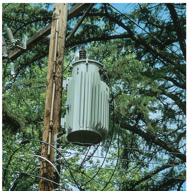
FIGURE 6.34 Energy losses in transmission are reduced by increasing the voltage, so the voltage of generated power is stepped up at the power plant. (A) These transformers, for example, might step up the voltage from tens to hundreds of thousands of volts. After a step-down transformer reduces the voltage at a substation, still another transformer (B) reduces the voltage to 120 V for transmission to three or four houses. a & b: ©McGraw-Hill Education/Bill Tillery, photographer
