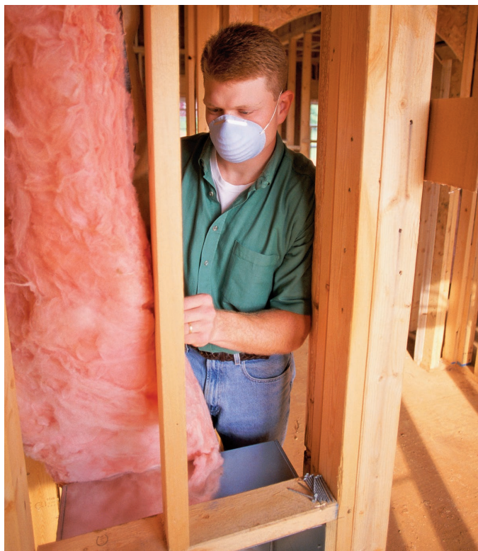
FIGURE 4.14 Fiberglass insulation is rated in terms of the R-value, a ratio of the conductivity of the material to its thickness.
