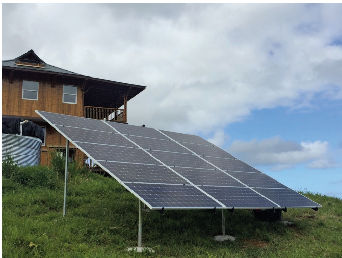
FIGURE 3.13 These 15 solar panels capture enough energy from the Sun in a single day to provide electricity for a typical house for several days. ©Timothy F. Slater
