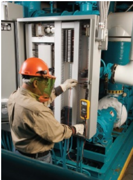
Figure 1-18 Testing for the presence of voltage.
