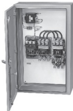
Figure 8-23 Wye-delta starter.
