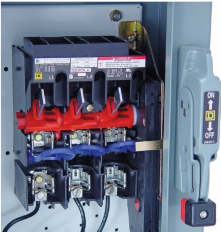
Figure 8-5 Disconnecting switch.
