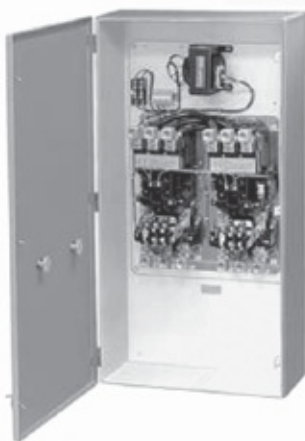
Figure 8-24 Typical part-winding starting circuit.
