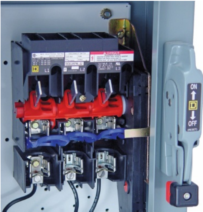
Figure 8-5 Disconnecting switch.
