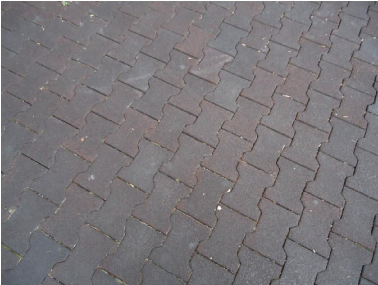
Figure 21.3 Interlocking Paving Bricks Made from Recycled Rubber.
