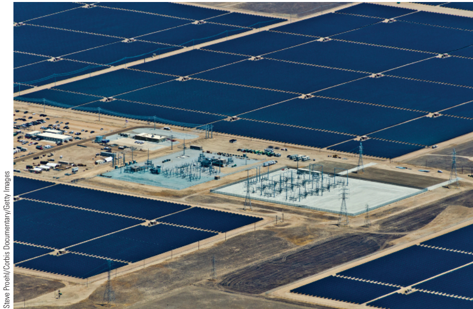
Figure 10.10 Topaz Solar Farm is one of the largest PV power stations in the world and can generate up to 550 MW.
