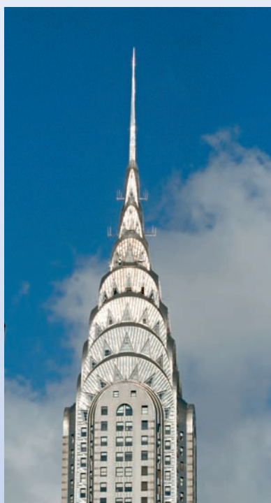
Built in New York in 1929, the Chrysler Building's stainless steel pinnacle has been cleaned only a few times. Despite the urban setting, the material shows few signs of corrosion.
