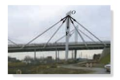
The four cable forces are all concurrent at point O on this bridge tower. Consequently they produce no resultant moment there, only a resultant force  $\mathbf{F}_R$ . Note that the designers have positioned the cables so that  $\mathbf{F}_R$  is directed *along* the bridge tower directly to the support, so that it does not cause any bending of the tower. (© Russell C. Hibbeler)
