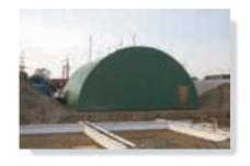
The resultant of a wind loading that is distributed on the front or side walls of this building must be calculated using integration in order to design the framework that holds the building together. (© Russell C. Hibbeler)
