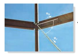
The angle  $\theta$  between the rope and the beam can be determined by formulating unit vectors along the beam and rope and then using the dot product  $\mathbf{u}_b \cdot \mathbf{u}_r = (1)(1) \cos \theta$ . (© Russell C. Hibbeler)
