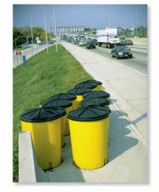
If an oncoming car strikes these crash barrels, the car's kinetic energy will be transformed into work, which causes the barrels, and to some extent the car, to be deformed. By knowing the amount of energy that can be absorbed by each barrel it is possible to design a crash cushion such as this. (© R.C. Hibbeler)
