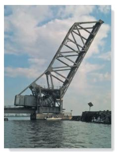
The counterweight on this bascule bridge does positive work as the bridge is lifted and thereby cancels the negative work done by the weight of the bridge. (© R.C. Hibbeler)
