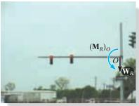
The weights of these traffic lights can be replaced by their equivalent resultant force  $W_R = W_1 + W_2$  and a couple moment  $(M_R)_O = W_1d_1 + W_2d_2$  at the support, O. In both cases the support must provide the same resistance to translation and rotation in order to keep the member in the horizontal position. (© Russell C. Hibbeler)
