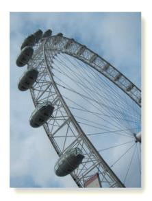
Riders on this Ferris wheel are subjected to curvilinear translation, since the gondolas move in a circular path, yet it always remains in the upright position. (© R.C. Hibbeler)
