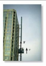
The power requirement of this hoist depends upon the vertical force  $\mathbf{F}$  that acts on the elevator and causes it to move upward. If the velocity of the elevator is  $\mathbf{v}$ , then the power output is  $P = \mathbf{F} \cdot \mathbf{v}$ . (© R.C. Hibbeler)
