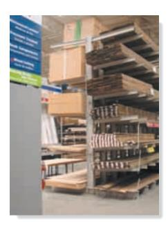
The shelving arms must be designed to resist the internal loading in the arms caused by the lumber. (© Russell C. Hibbeler)
