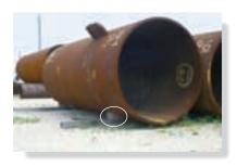
Wedges are often used to adjust the elevation of structural or mechanical parts. Also, they provide stability for objects such as this pipe. (© Russell C. Hibbeler)
