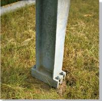
During impact the columns of many highway signs are intended to break out of their supports and easily collapse at their joints. This is shown by the slotted connections at their base and the breaks at the column's midsection. (© R.C. Hibbeler)
