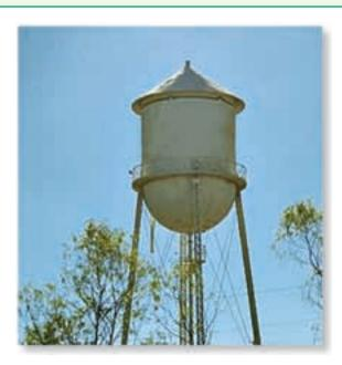
The center of gravity of this water tank can be determined by dividing it into composite parts and applying Eqs. 9–6. (© Russell C. Hibbeler)
