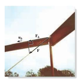
The projection of the cable force  $\mathbf{F}$  along the beam can be determined by first finding the unit vector  $\mathbf{u}_b$  that defines this direction. Then apply the dot product,  $F_b = \mathbf{F} \cdot \mathbf{u}_b$ . (© Russell C. Hibbeler)
