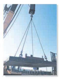
Cartesian vector analysis provides a convenient method for finding both the resultant force and its components in three dimensions. (© Russell C. Hibbeler)
