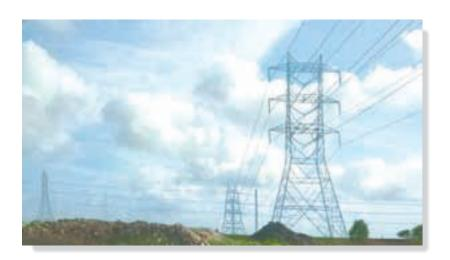
Electrical transmission towers must be designed to support the weights of the suspended power lines. The weight and length of the cables can be determined since they each form a catenary curve. (© Russell C. Hibbeler)
