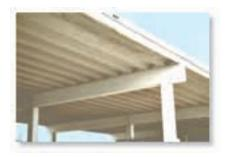
This concrete beam is used to support the deck. Its size and the placement of steel reinforcement within it can be determined once the shear and moment diagrams have been established. (© Russell C. Hibbeler)
