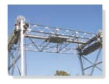
The use of metal gusset plates in the construction of these Warren trusses is clearly evident. (© Russell C. Hibbeler)
