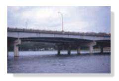
To save on material and thereby produce an efficient design, these beams, also called girders, have been tapered, since the internal moment in the beam will be larger at the supports, or piers, than at the center of the span. (© Russell C. Hibbeler)
