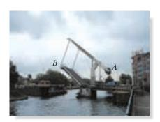
The counterweight at A balances the weight of the deck B of this simple lift bridge. By applying the method of potential energy we can analyze the equilibrium state of the bridge. (© Russell C. Hibbeler)
