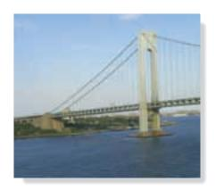
The cables of the suspension bridge exert very large forces on the tower and the foundation block which have to be accounted for in their design. (© Russell C. Hibbeler)
