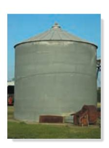
The amount of material used on this storage building can be estimated by using the first theorem of Pappus and Guldinus to determine its surface area. (© Russell C. Hibbeler)
