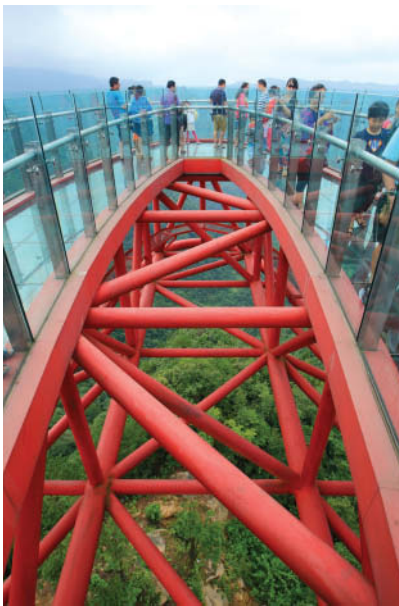
A space truss is incorporated into the world's longest glass skywalk which is located in Huangshi National Forest Park in Chongqing, China.
