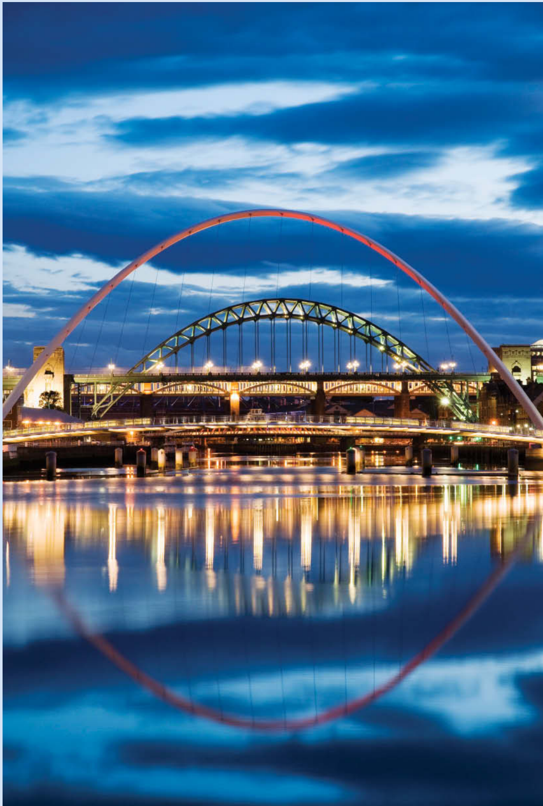
This view of the River Tyne in the United Kingdom shows a variety of structures, including the Gateshead Millennium Bridge (closest to the camera). This award-winning bridge can rotate about a horizontal axis along its span to allow ships to pass underneath.
