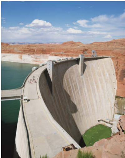
Glen Canyon Dam at Lake Powell, Arizona
