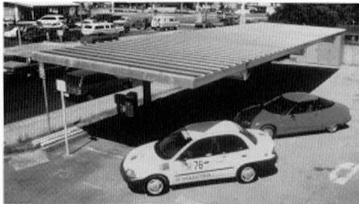
Modules integrated into the roof of a parking structure provide both power and protection for electric vehicles.
