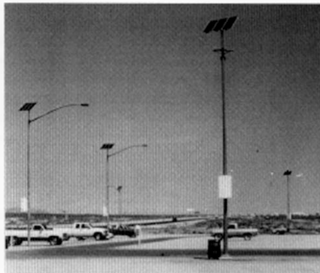
No wires—underground or overground—were needed to light this parking area. Each streetlamp has its own solar module providing its electricity.
