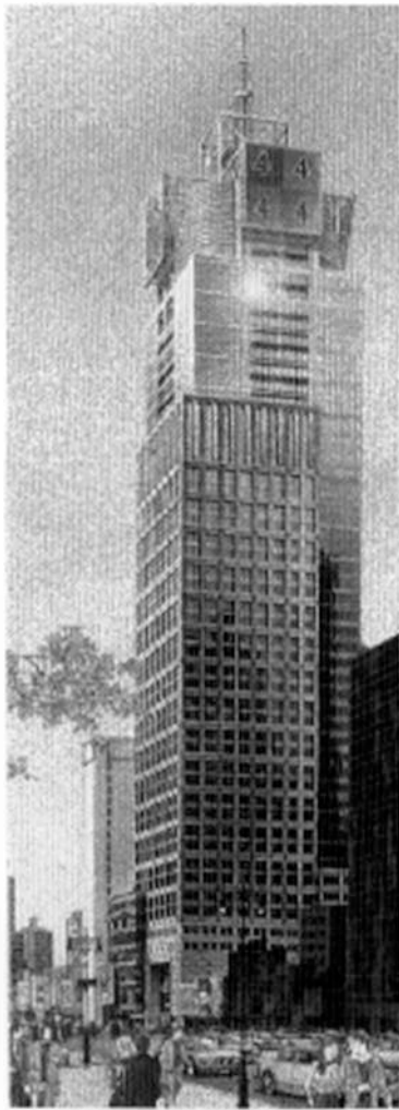
The first major American commercial building to use photovoltaics as part of its facade is 4 Times Square.
