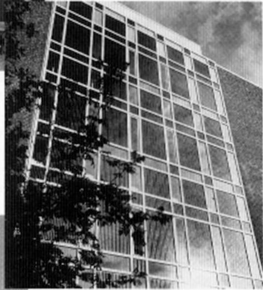
Right: Flachglas' first installation that integrated solar cells into a building's facade. Here photovoltaics replaced the vertical glass on the south side of the structure.
