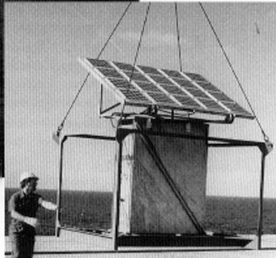
Securing a photovoltaic array on an oil platform in the Gulf of Mexico.
