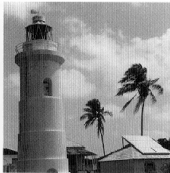
Today, solar cells power the lights in almost every lighthouse run by the Coast Guard.
