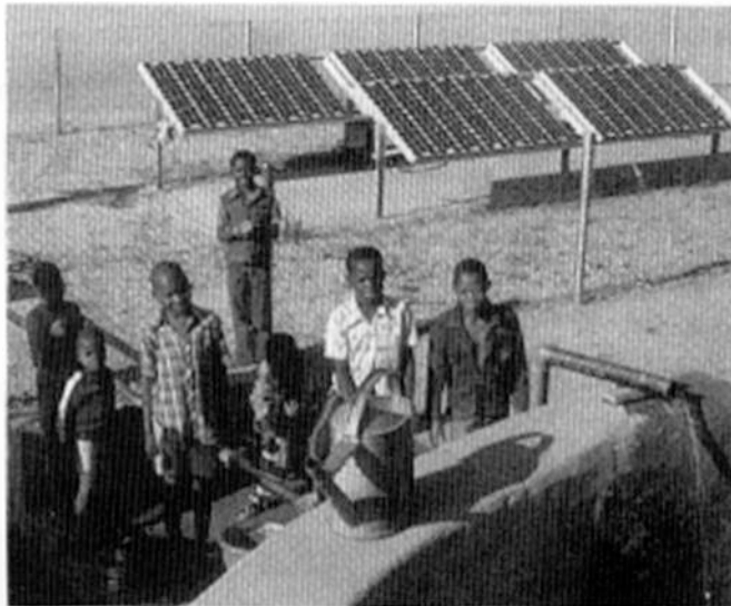
Young Malian boys watch a photovoltaic-driven pump fill their village's formerly dry cistern with water.
