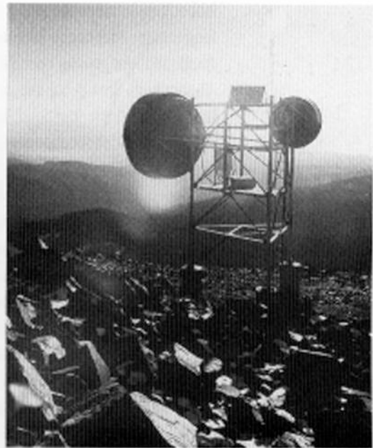
A view of the Hunts Mesa solar-run repeater, with a panorama of the rugged landscape that made its placement a necessity to provide Mexican Hat, Utah, with long-distance phone service.
