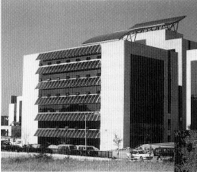
Left: Photovoltaic shades can help control the amount of solar heat entering a building, thus reducing the electricity consumed by air conditioning.
