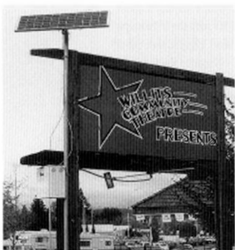
A prepackaged stand-alone photovoltaic unit lights this sign at night.
