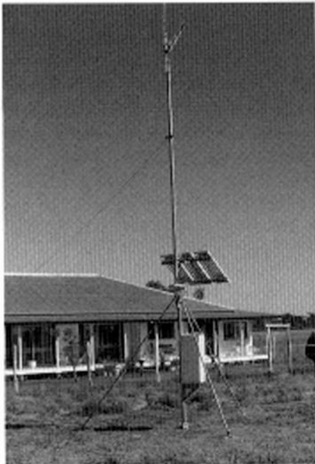
Photovoltaics allows this isolated Australian homestead to communicate with the outside world as easily as urban dwellers.
