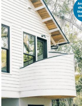
The trim is made of fly-ash (a byproduct of burning coal) combined with polymers, making it more durable than wood. Designed to withstand winds of
