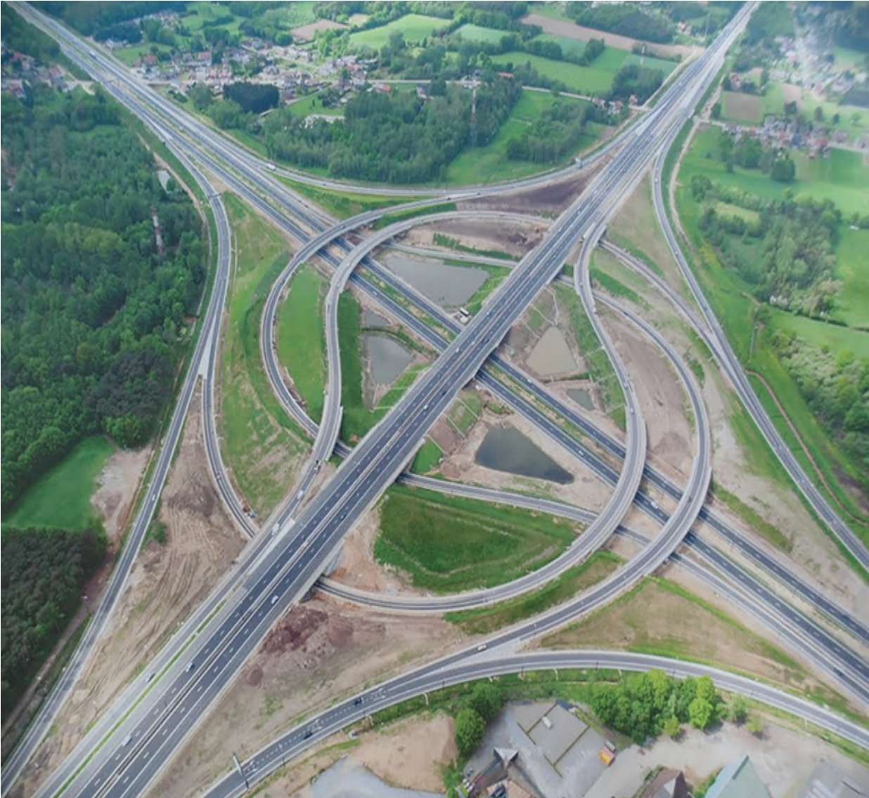
Figure 8.3 The highway interchange in Lummen, Belgium, redesigned between 2008 and 2012. Twelve new bridges, some weighing 8,000 tons, were built and moved around. This elegant engineering solution inspired our interviewees and can be beautiful, just like a work of art. Photo courtesy of Davy Govaert.
