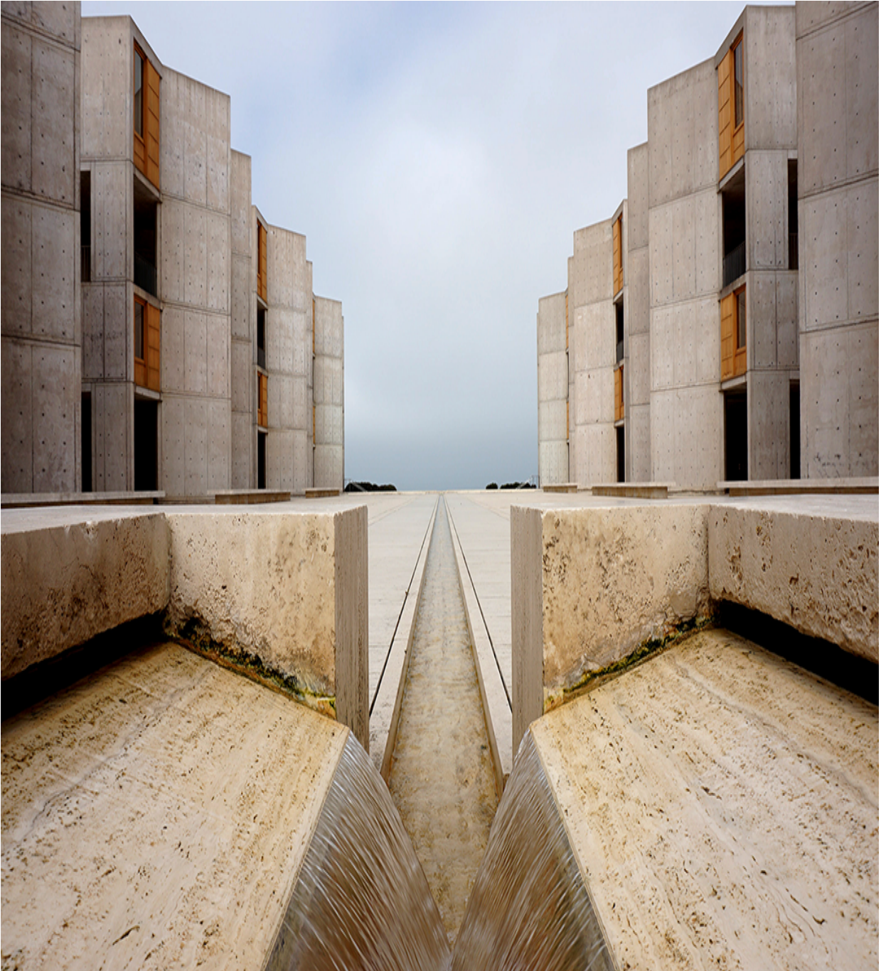
Figure 7.6 The Salk Institute courtyard showcasing a mirrored structure containing strategically placed laboratories, utilities, office spaces overlooking the Pacific Ocean, and study areas. Photo courtesy of Adam Bignell, Unsplash.
