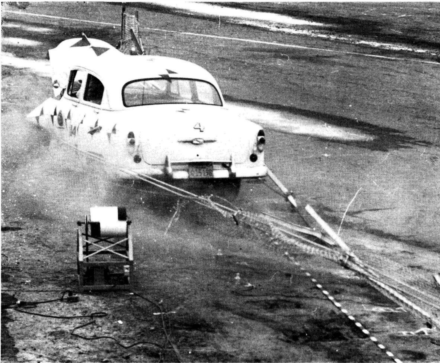
Chain-link fence snares hurtling vehicle while cables cut in above and below front wheel, keeping car in own lane.
