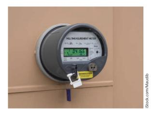
Figure 8-6 A single-use, plastic security seal
