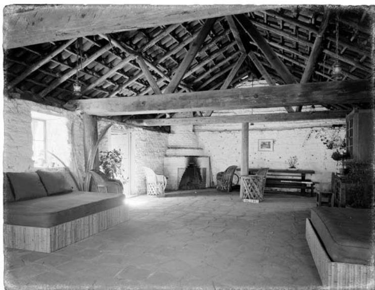
Leaving the vigas (beams) and latillas (branches) exposed makes for a rich, warm ceiling.
