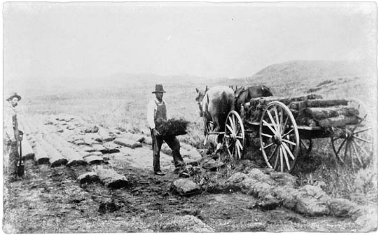
Sod strips were cut from the prairie, loaded on a wagon, and brought to the building site.
