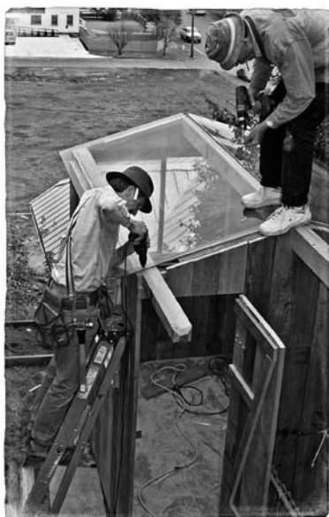
Plexiglas makes a good roof covering and lets in lots of sunlight.
