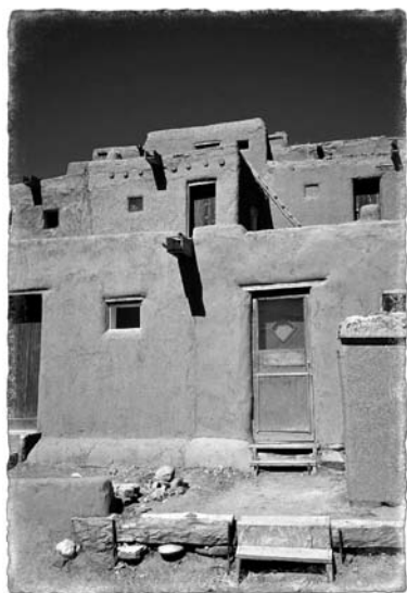
Houses built from adobe, Mother Earth, are home to billions of people across the globe. The Taos Pueblo in New Mexico has been occupied by Native people for many centuries.
