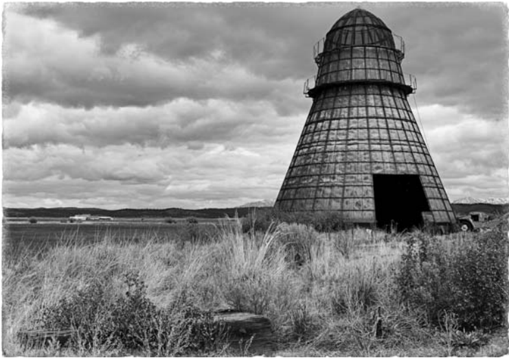
The lumber mills burned a good part of every tree in wigwam burners.
