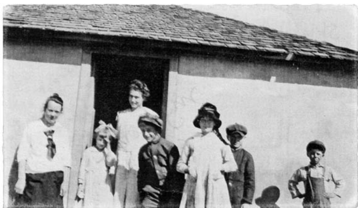
My mother with her students in front of their straw bale schoolhouse in 1917. It has been stuccoed with a clay-lime mixture.
