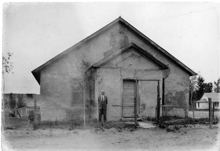
This straw bale church was built in 1928 and still serves the community in the small village of Arthur, Nebraska.
