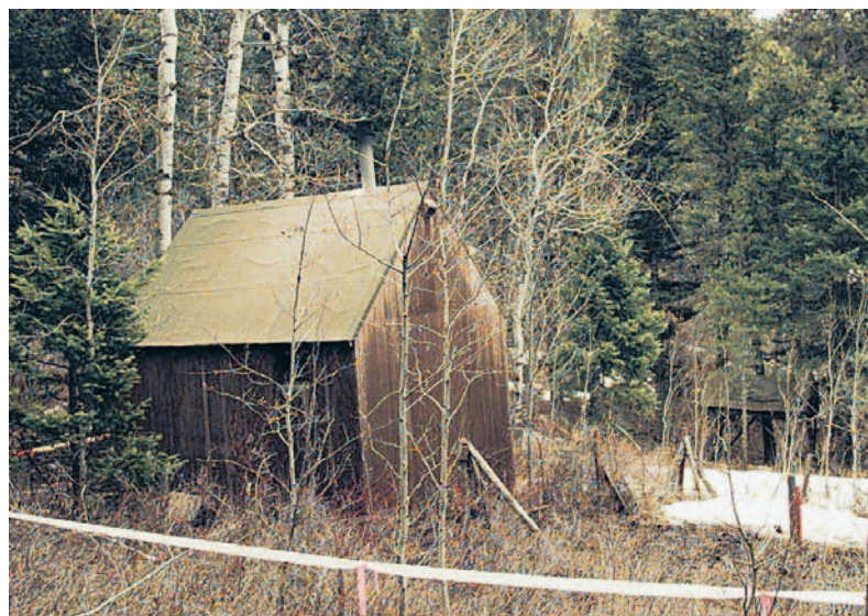
The cabin where Kaczynski lived in Lincoln, Mont., had no electricity or running water.
