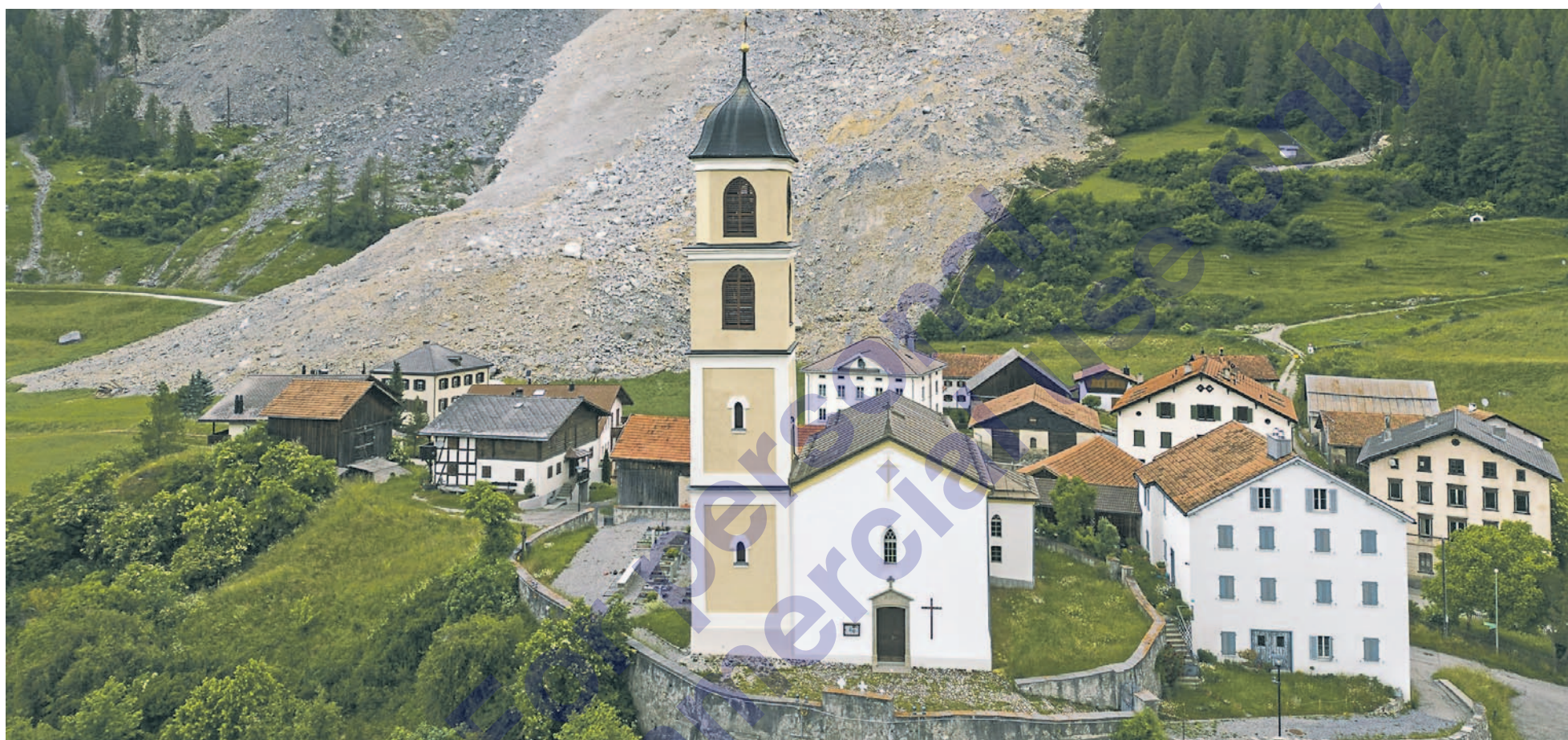
FALLING ROCK: A huge mass of rock slid down a mountain above Brienz, Switzerland, early Friday and stopped just short of the village. Residents had been evacuated last month.
