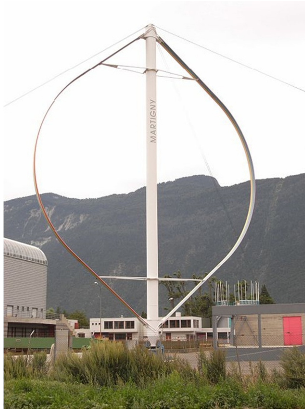
FIG. 6.9 Darrieus type vertical axis wind turbine. Source: Wikipedia.
