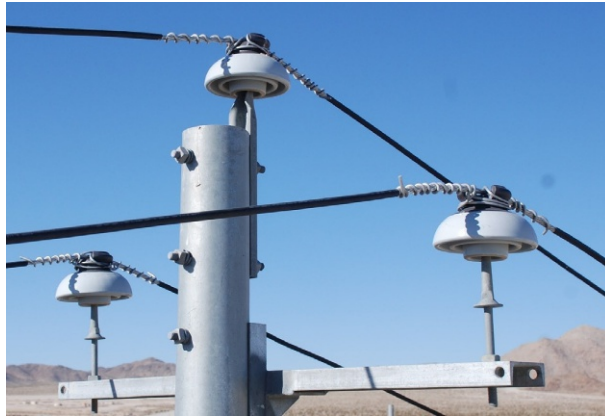
FIG. 3.21 Pin type insulator. Source: Wikipedia.
