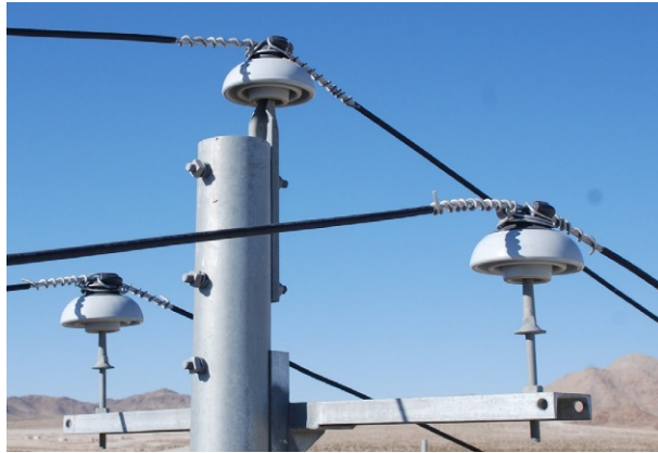
FIG. 3.21 Pin type insulator. Source: Wikipedia.
