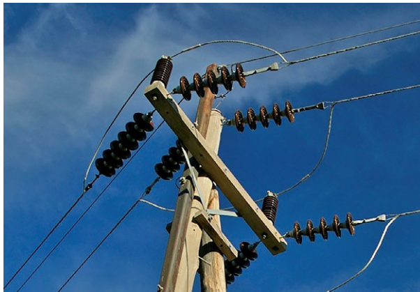
FIG. 3.23 Strain insulator. Source: Wikipedia.
