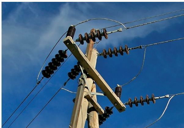
FIG. 3.23 Strain insulator. Source: Wikipedia.
