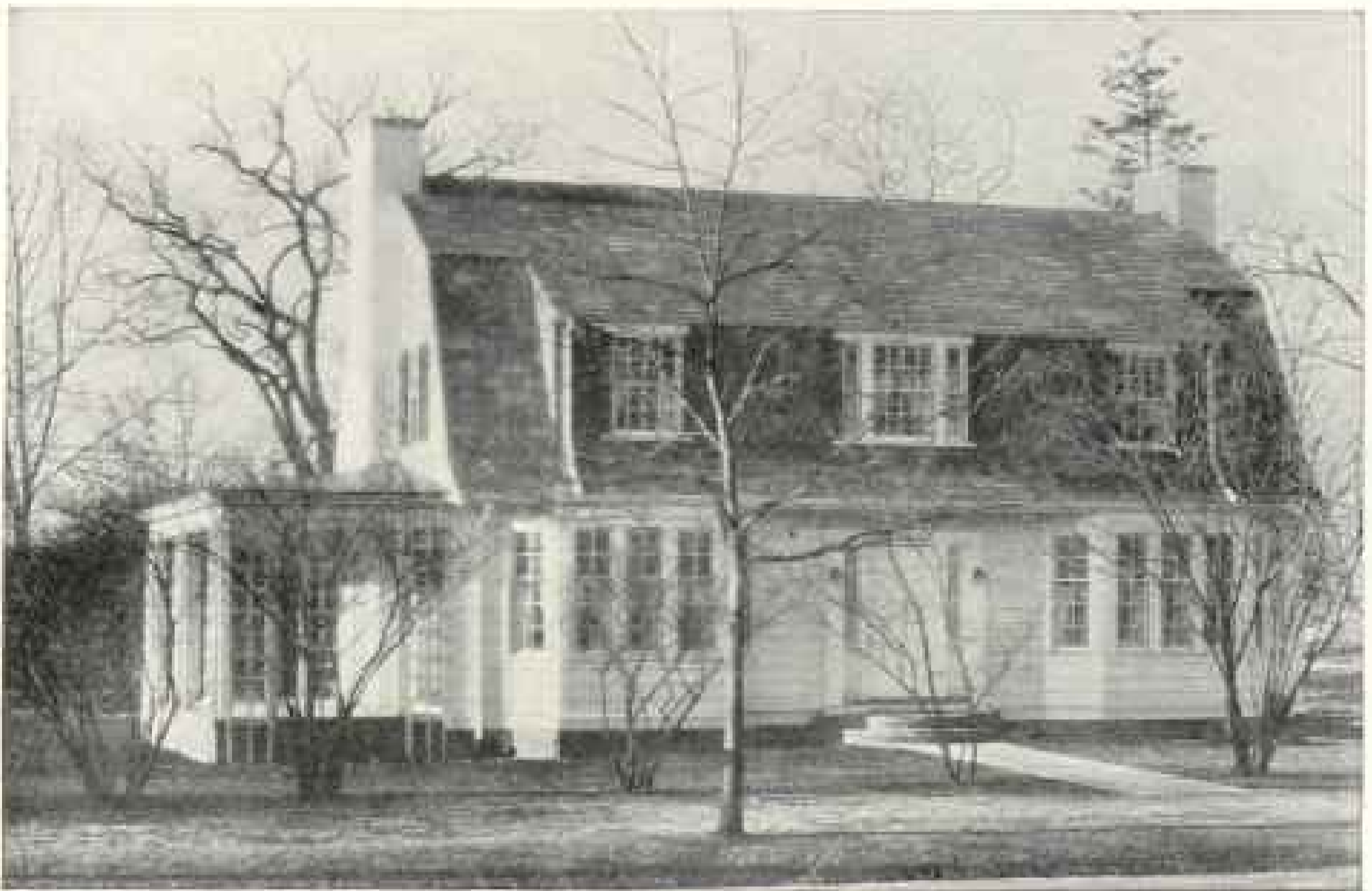
House on Fresh Pond Parkway, Cambridge, Mass. Charles R. Green, Architect, Boston, Mass.
