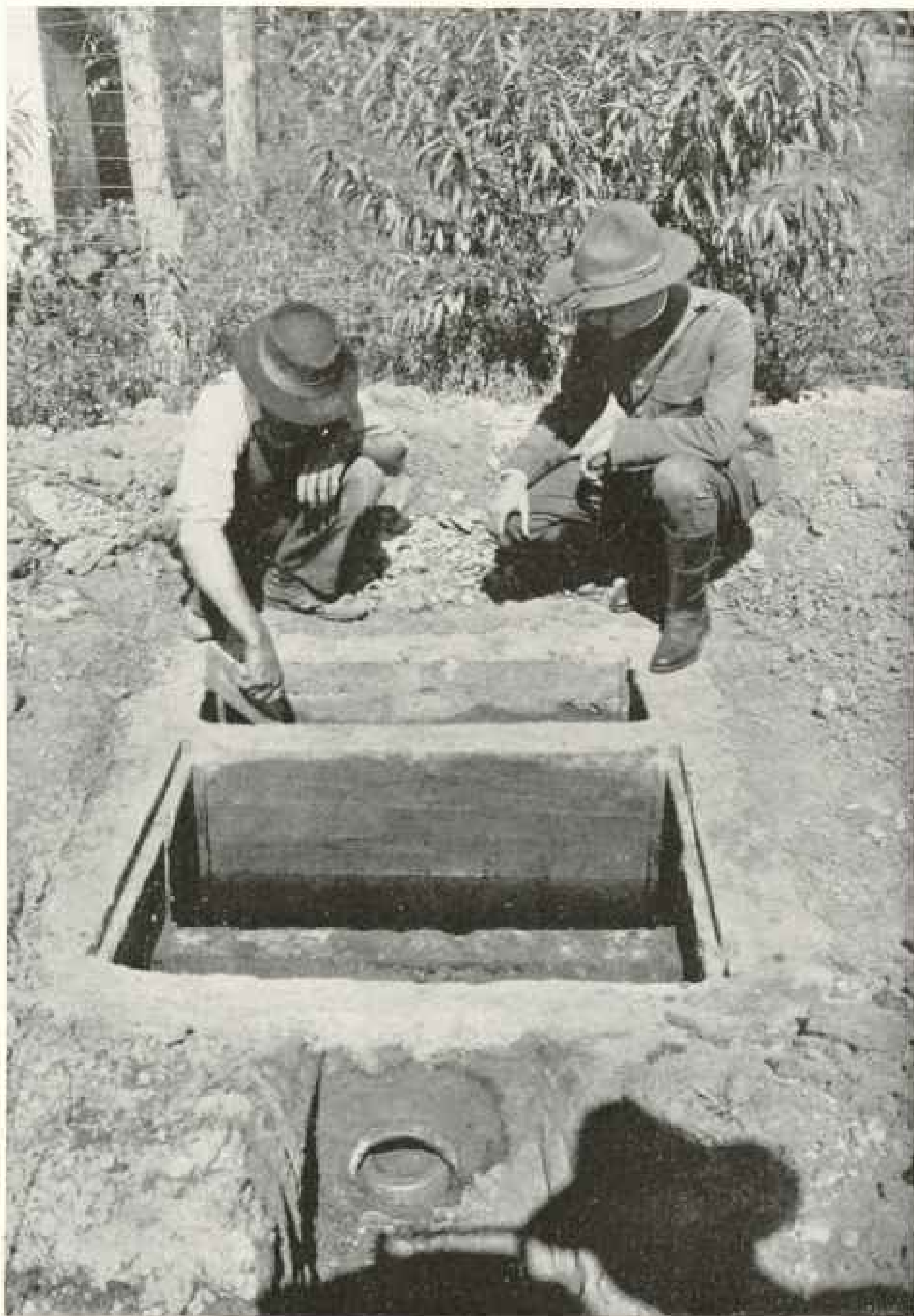
CONSTRUCTION OF SANITARY PRIVY, SHOWING DOUBLE CHAMBERS AND EXIT OF DRAIN: EXTRA CANTONMENT ZONE, CAMP ZACHARY TAYLOR (SEE PAGE 277)
