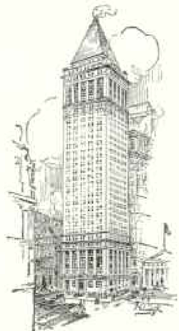
Bankers Trust Company Building
