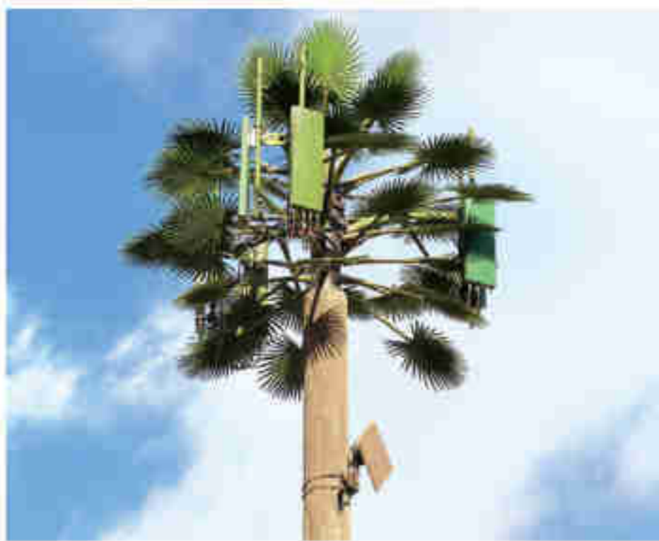
The fruit of the palm: antenna panels.
