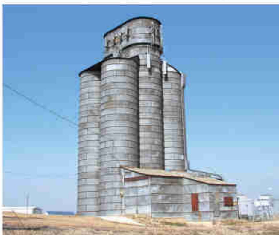
Former sugar silos now hold phone gear.
