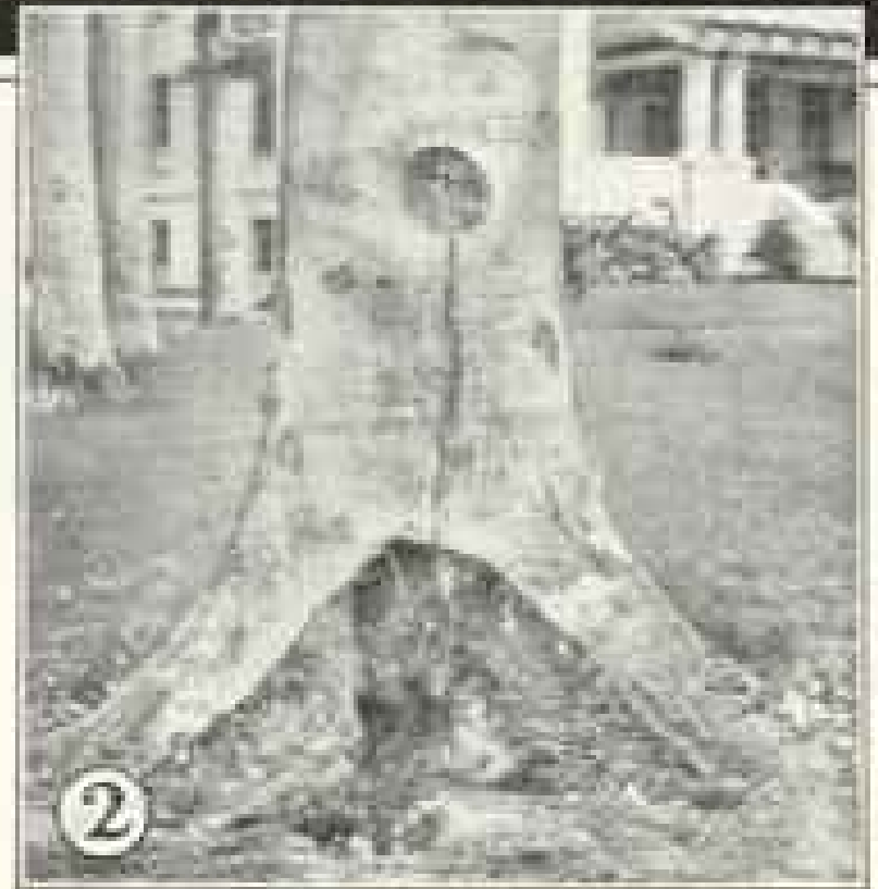
2 Crude patch removed—showing accuracy and regional decay.
