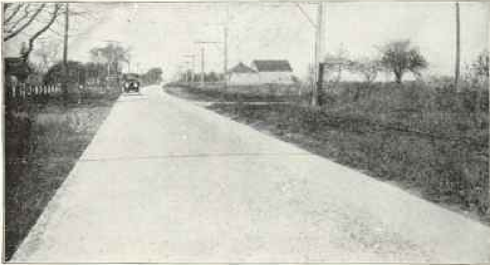
Lake Shore Concrete Road Near Kenosha, Wis., Built for the State Highway Department by G. E. Wade, of Kenosha, in 1915
