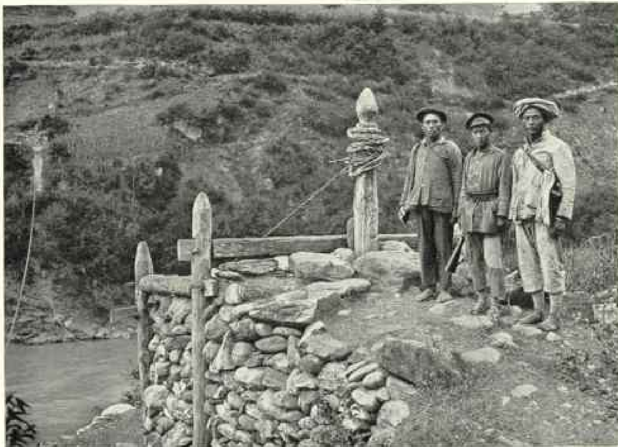
THE ROPE BRIDGE OVER THE MEKONG AT LOTA IS WELL ANCHORED
