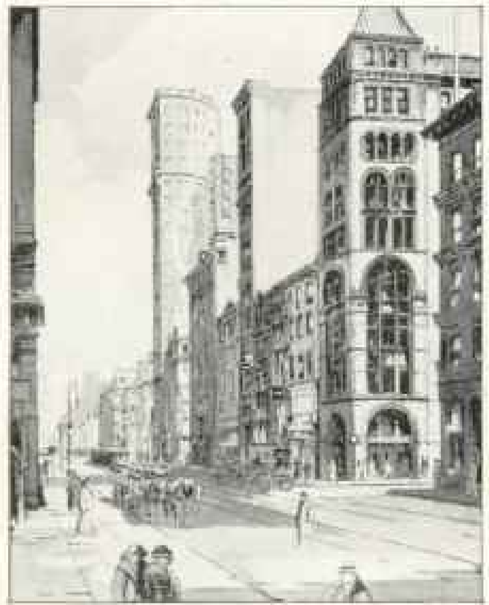
The same scene after the overhead wires were replaced by underground cables
