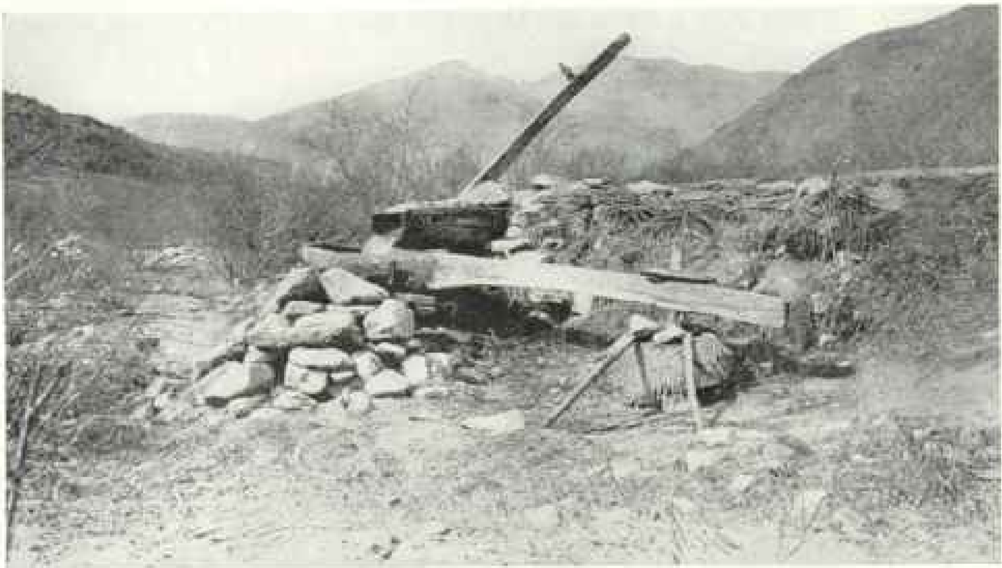
AN HYDRAULIC HAMMER À LA KOREA, USED IN POUNDING GRAIN
