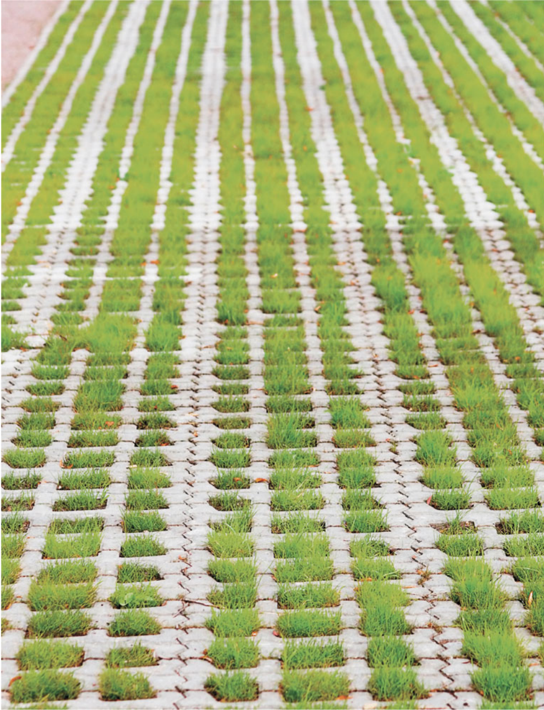
Permeable pavers can have small gaps and be installed like brick or they can have larger gaps where grass can grow through.
