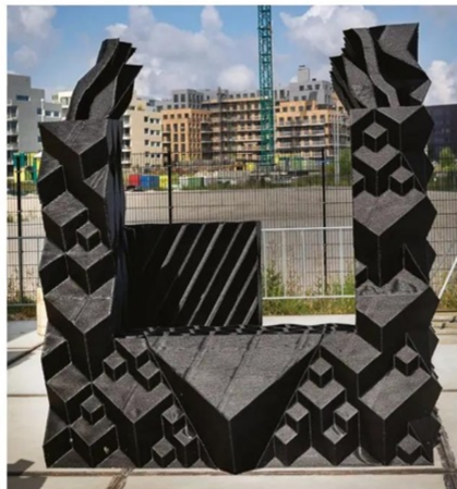
The Canal House in Amsterdam is a continually evolving building, adapted with new 3D-printed parts
