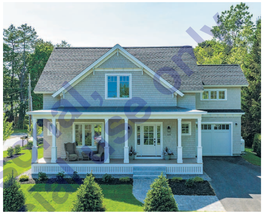
449 Black Point Road Scarborough, Maine
