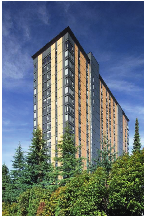
Figure 5. Brock Commons Tallwood House (photo by Michael Elkan and courtesy of Acton Ostry Architects).
