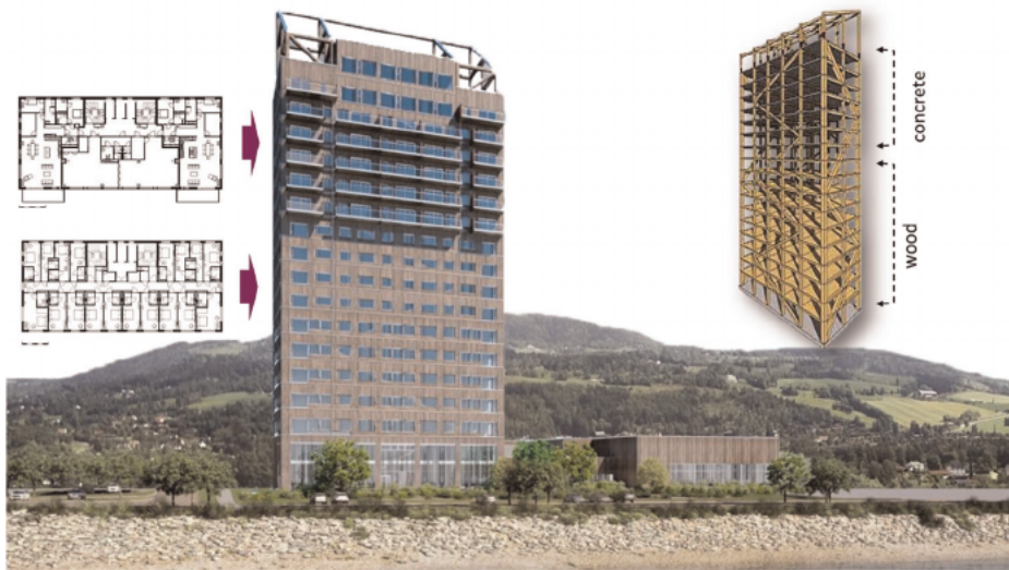
Figure 4. The “Mjøsa” tower in Norway.
