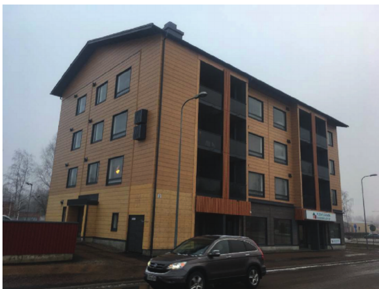
Figure 7. A four-story log apartment, Finland (photo by Hüseyin Emre Ilgin).
