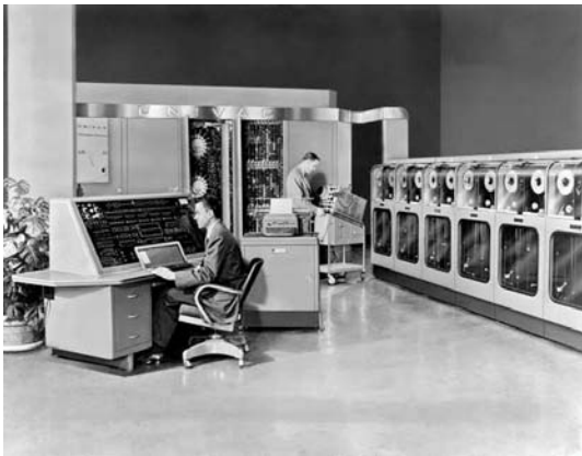
Figure 8.2. Above is a picture of the first ever computer bureau or commercial computer. It was considered a mathematical genius that was eight feet tall. It was able to classify citizens in a sixth of a second according to their income, employment, birthplace, age group, residence, education, and sex marital status.
