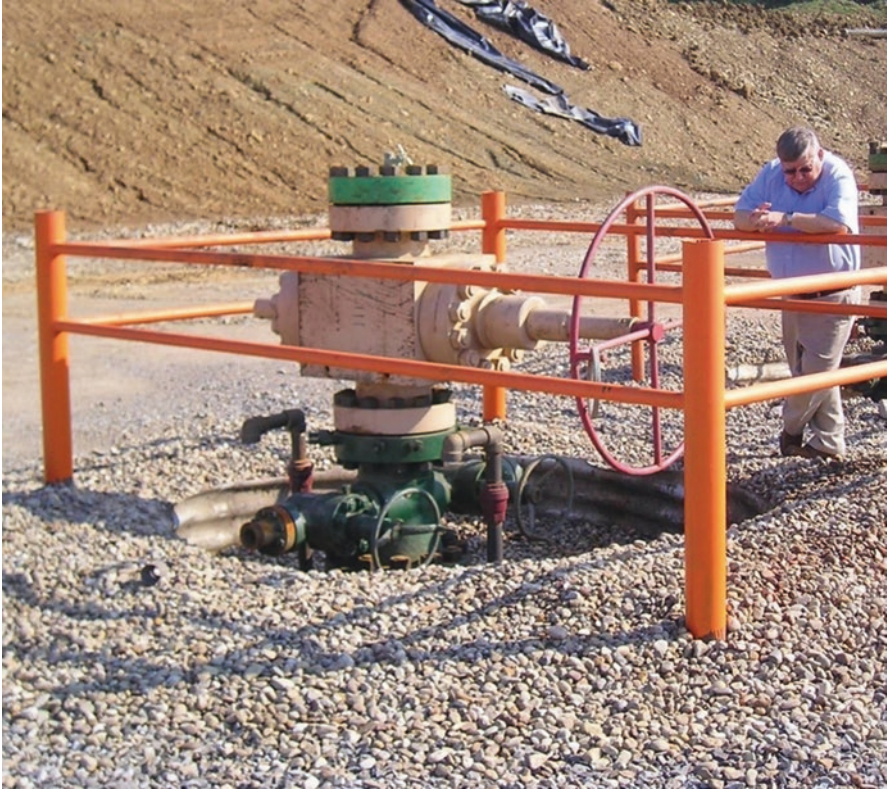
Fig. 2.4 A massive wellhead known as a frack gate on a Marcellus Shale well in Pennsylvania with geologist Bill Schuller standing nearby for scale. (Photographed in 2011 by Dan Soeder)
