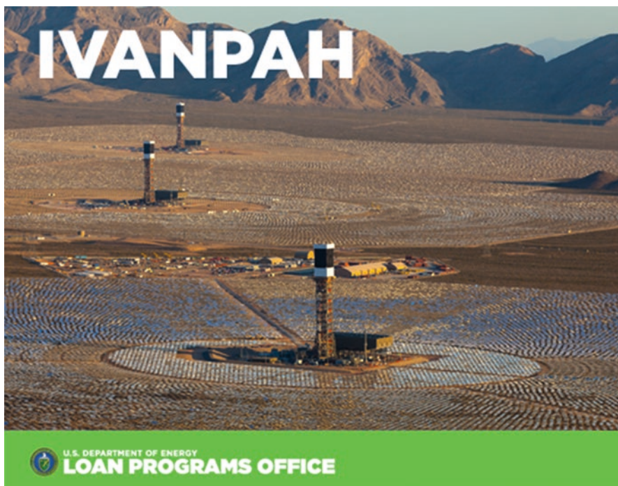
Fig. 9.5 Solar power towers surrounded by mirrors at Ivanpah Dry Lake, California. (Photo: U.S. Department of Energy)
