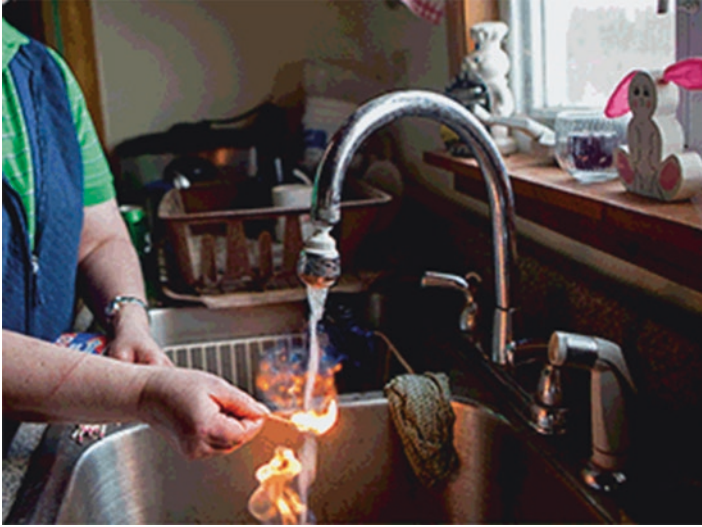
Fig. 1.1 A flaming kitchen faucet caused by natural gas entering a domestic water supply well in Pennsylvania. Images like this have become linked to environmental concerns about fracking. (Photo copyright Getty Images; used under license)
