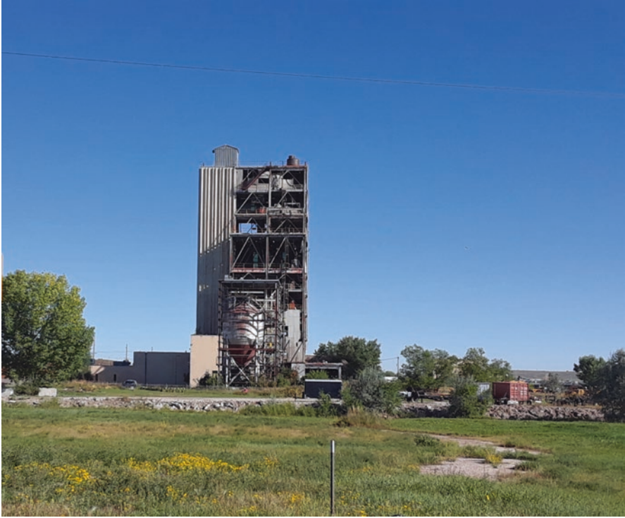
Fig. 4.2 Abandoned, 1980s era coal-to-liquids (CTL) pilot plant south of Rapid City, SD. (Photographed in 2019 by Dan Soeder)
