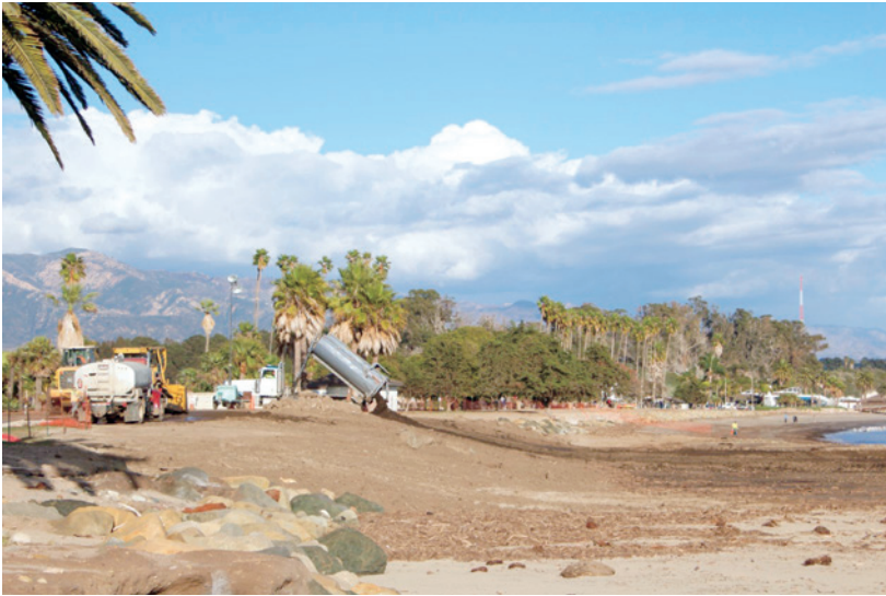
FIG 8.4 Ordinarily, a mud-nourished beach would be considered a failed project. In 2018, mud was poured on purpose onto Goleta Beach in California, in an emergency case. A mudflow had smashed into the city of Santa Barbara after forest fires removed stabilizing vegetation from nearby mountain slopes. The mud (with toxins, like oil) had to be removed from the city streets, and the beach and ocean provided a convenient dumping site. Photo © Vanessa Lytle.
