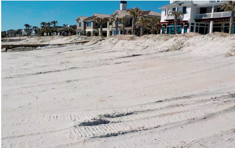
FIG 8.6 The scraped beach and dune on Ponte Vedra Beach, Florida. Sand was bulldozed up from the lower beach to elevate the upper beach, in order to provide storm protection for private homes. The problem is that this process narrows the public's beach. The property owners responsible for the scraping were fined $234,000 by the state. Photo courtesy of the Florida Department of Environmental Protection.
