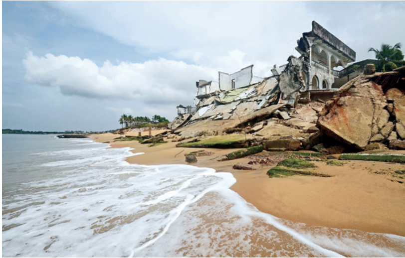
FIG 9.3 The remnants of the town of Grand-Lahou near the Lakka Beach Resort in Sierra Leone. The erosion here has been caused almost entirely by nearby mining activities, which started in 2013. The destroyed buildings act as a seawall, slowing down erosion. Grand-Lahou was moved 10 miles (16 km) inland—an example of managed retreat. Photo © Tommy Trenchard.
