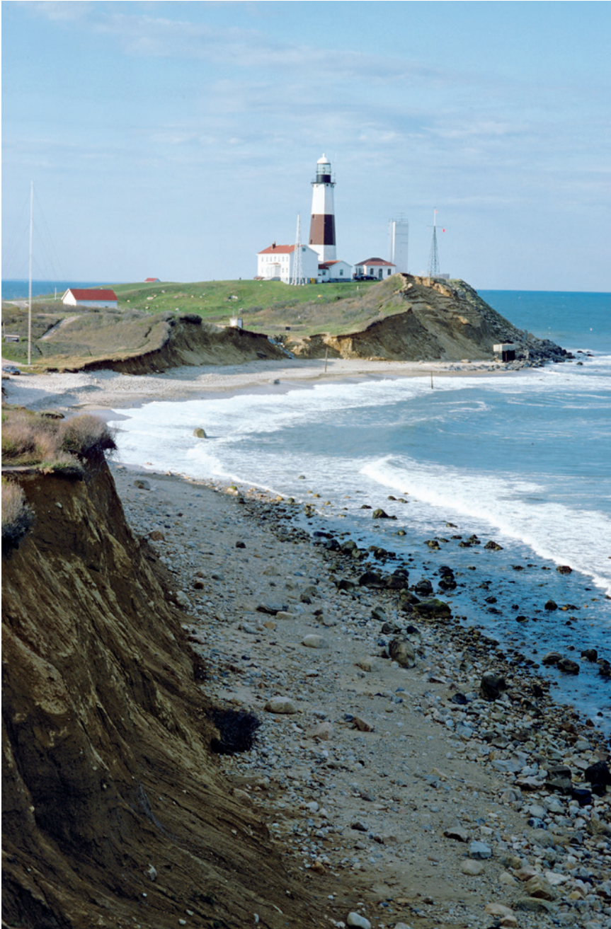
FIG 10.4 Lighthouse on Long Island, New York, on top of a rapidly eroding bluff that supplies sediment to local beaches. Eventually, in order to save it, the lighthouse may have to be moved back like the Cape Hatteras lighthouse in North Carolina was. Photo © Miles Hayes.
