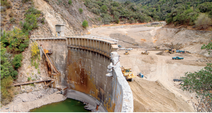
FIG 5.1 The removal of the San Clemente Dam near Monterey, California, in 2015, revealed that the impoundment was filled with sands and gravels that had accumulated behind the dam over a period of about ninety years. The fill rendered the dam useless and presented a flood and surge hazard if the dam failed. A good guess is that most of the fill was hauled away, rather than being reintroduced to feed the downstream channel and ultimately the shore. Photo © Luke Gianni, California American Water.
