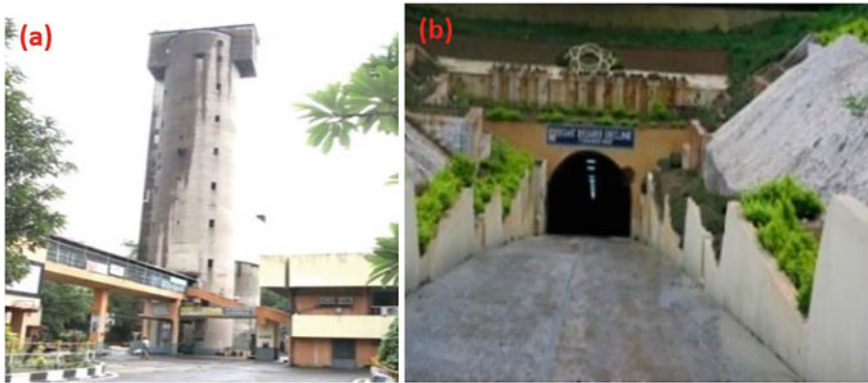
Fig. 2.5 Access to underground mines of uranium in Singhbhum district of India a shaft and b decline ( https://www.ucil.co.in , Accessed in March 2021)
