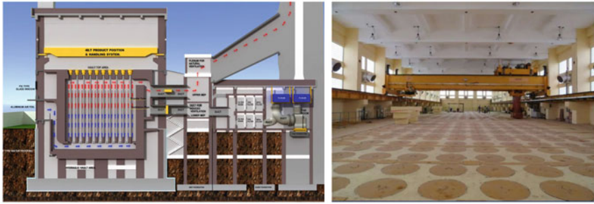
Fig. 8.25 Schematic and actual view of VWSF, Kalpakkam, India
