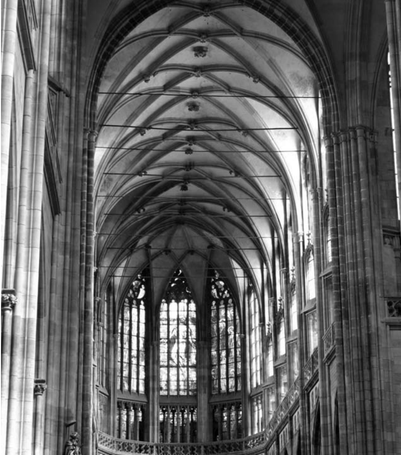
Iron tie-rods counteract the outward thrust of the vaults at Prague cathedral. (Photo: Janusz Leszczynski.)
