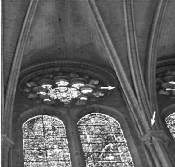
Stilting of the semicircular clerestory arches in the nave at Chartres. The springing points are indicated with white arrows. (Photo: Alex Rowbotham/AGRFoto.)
