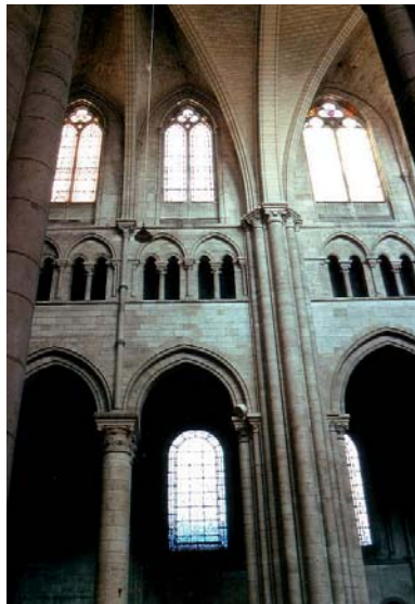
The nave elevation of Sens Cathedral, the construction of which began in the 1140s. (Note that the clerestory was remodelled in the thirteenth century.)
