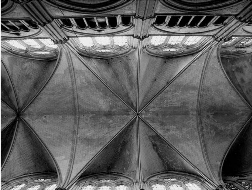
The sexpartite vault – and how it looks at Bourges Cathedral. (Photo: James Mitchell.)
