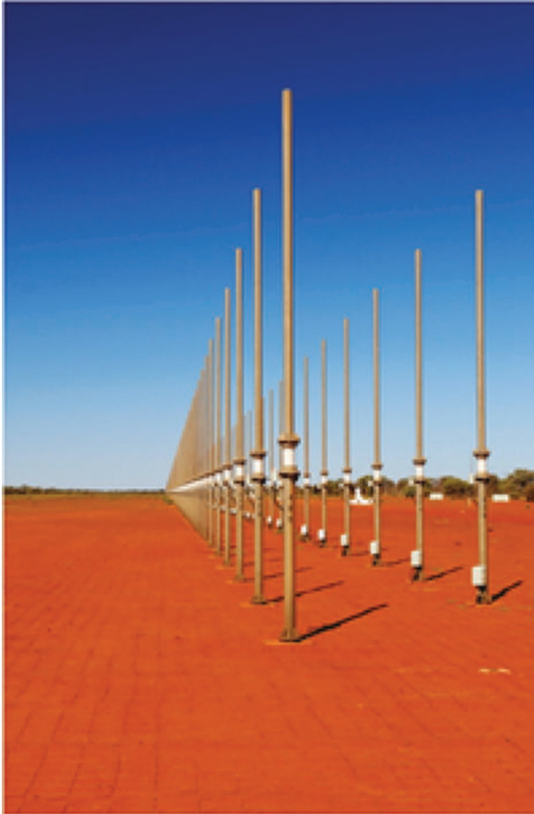
Figure 4.8 The JORN radar antenna
